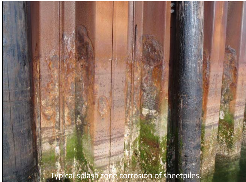
Figure 2 – Splash Zone Corrosion of Sheetpile – July 2011
