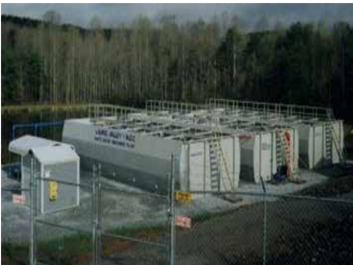
Example Multi-Unit Package Treatment Plant (Photo from: http://www.purestream.com )
