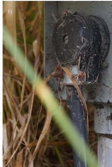
Photograph 25: Outbuilding feeder plug with spider webs and plant debris accumulation.
