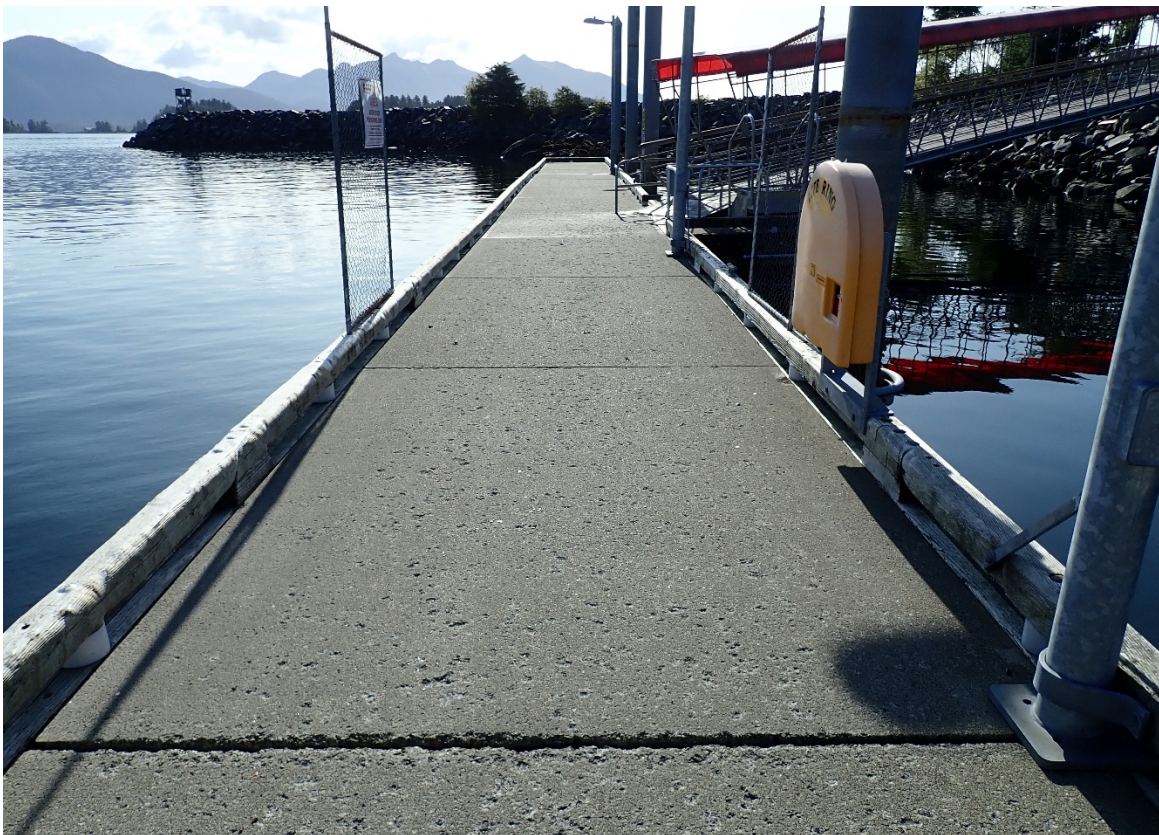
Photograph 4: View of topside scaling on south section of Lightering Float.
