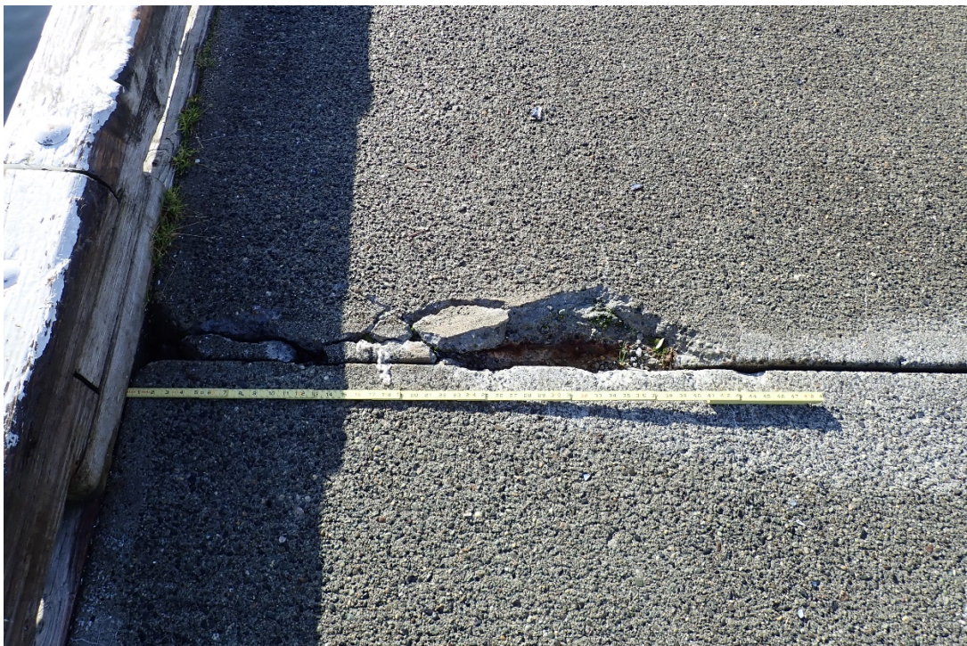
Photograph 2: Close up view of spall with exposed reinforcement on north edge of Float 6.
