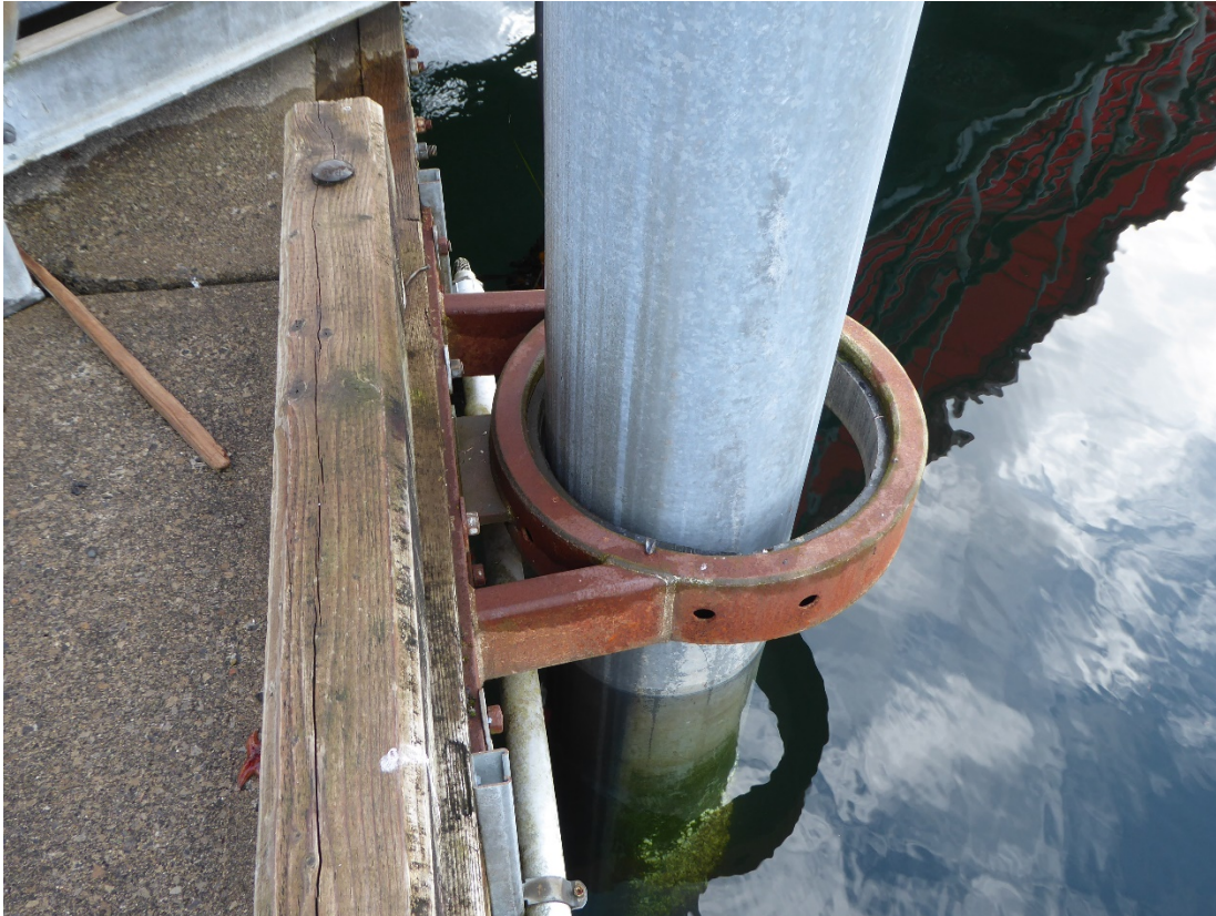
Photograph 13: Moderate corrosion at pile guide.
