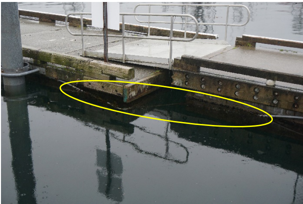
Photograph 16: Unfastened conduit.
