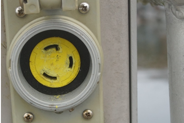
Photograph 22: Worn receptacle.
