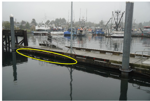
Photograph 17: Unfastened conduit.
