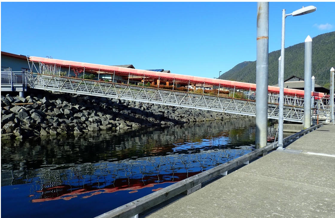
Photograph 14: View of South Gangway with light surface corrosion on rails.
