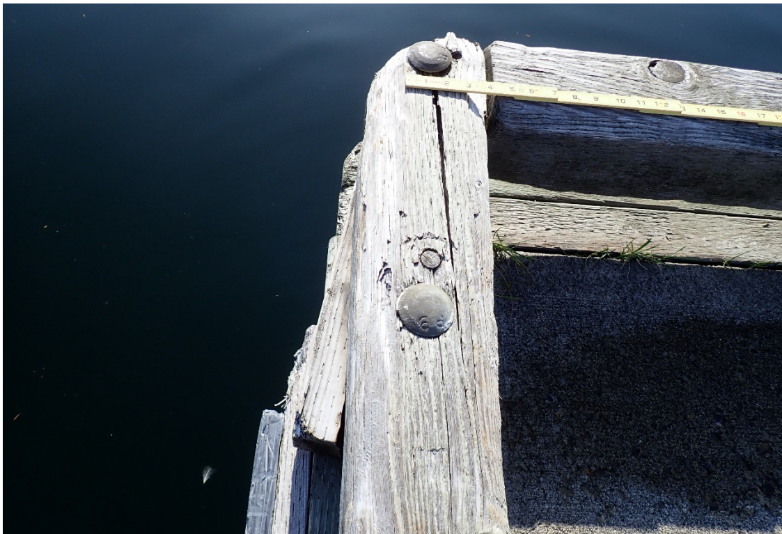
Photograph 6: View of the split upper rail and chock at the southeast corner of Float 22.
