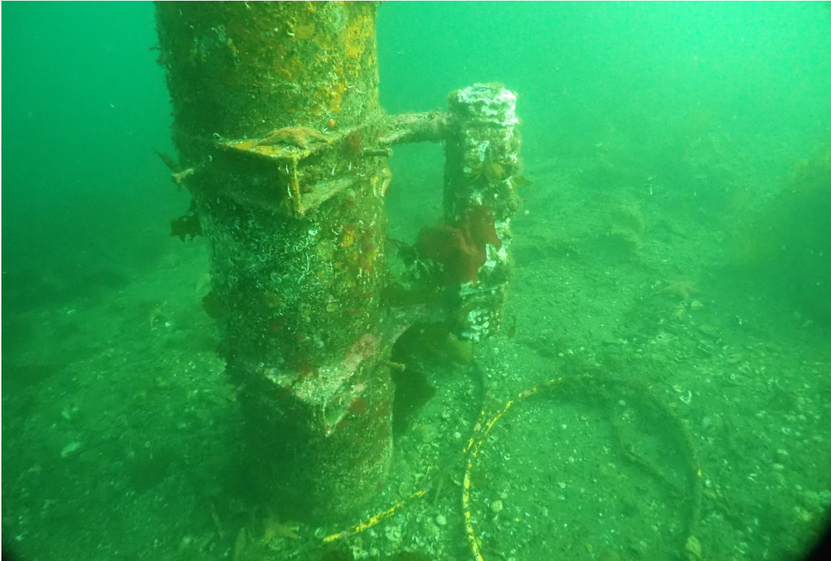
Photograph 11: Underwater view of typical anode and bracket on a Lightering Float pile.
