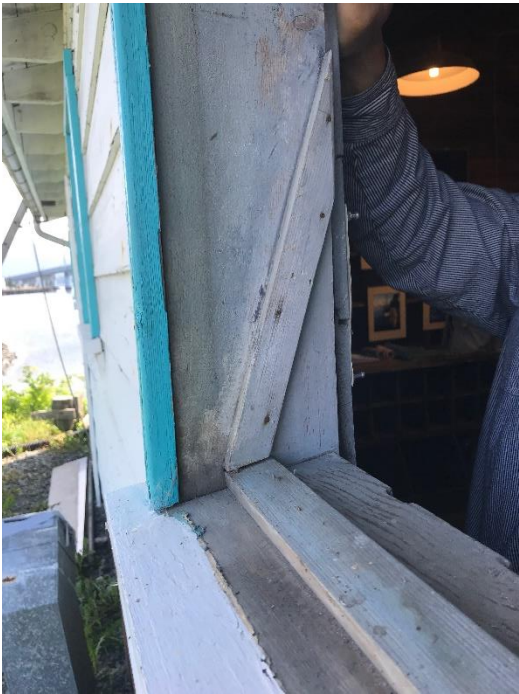
Detail of original window design— diagonal stops allow the sash to be tilted inward without the use of hinges. (07/01/2019)
