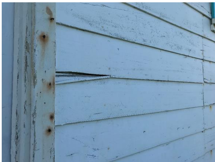
Detail of weathering and damage on Northeast wall (07/01/2019)
