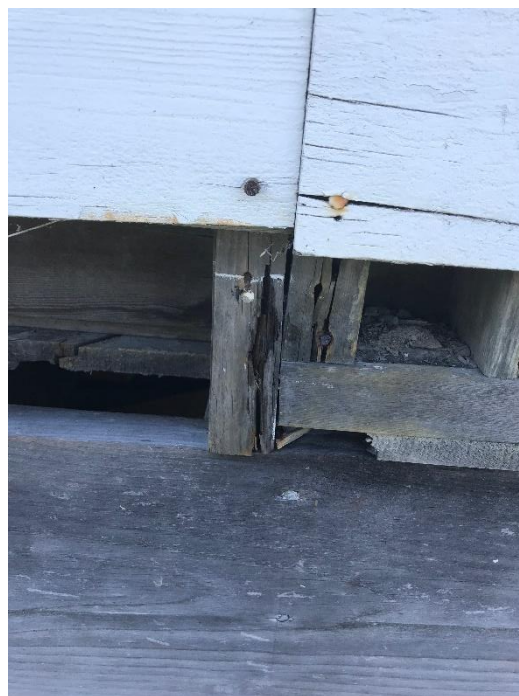
Detail of weathering on Northeast wall and studs (07/01/2019)
