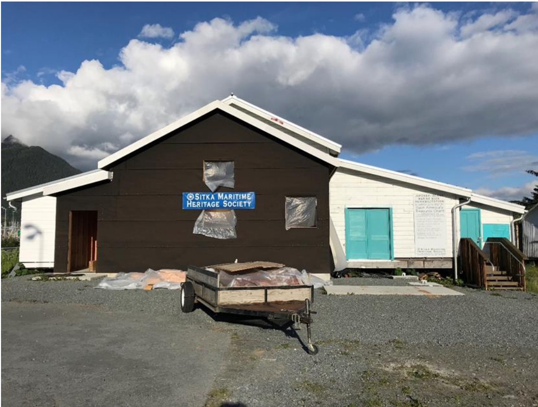
West view of the boathouse with new entry addition. Addition is covered and tar paper and has only rough openings for windows and doors. (06/24/2019)
