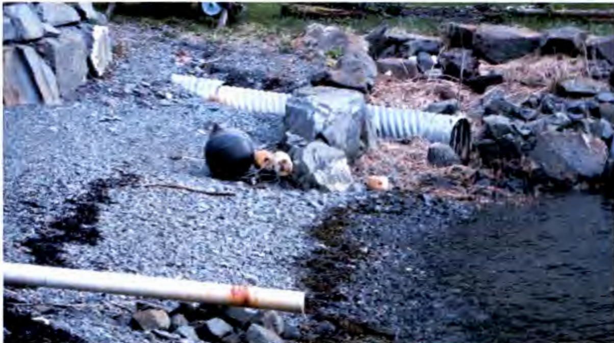
Outlet of Culvert just after a 9.1' High Tide. Wetted Edge and Scum line Showing Extent of Tide reaching the Outlet of the Culvert.
