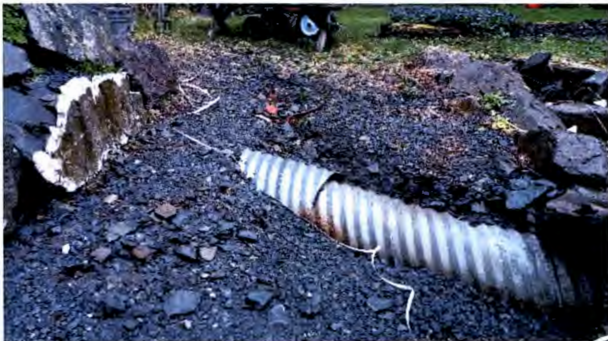
Photo of Seam Between Two Culverts on Downstream Side. Some Surface Erosion from Overland Flow or Wave Action above Lower End of Larger Culvert. High Tide Line (12.5') approximately at Margin of Grass and Gravel Above Culverts.
