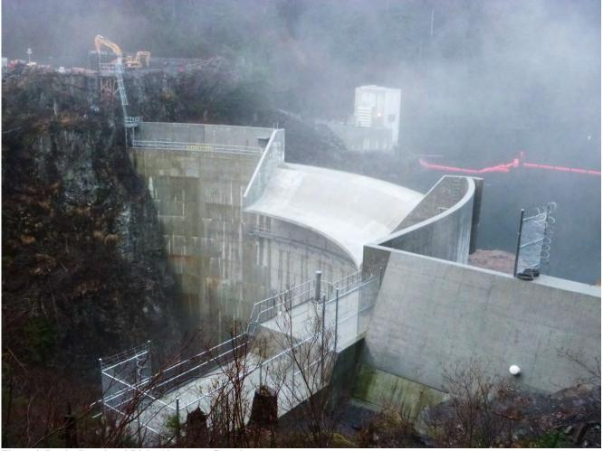
Figure 2. Intake Portal and Right Abutment, Complete.
