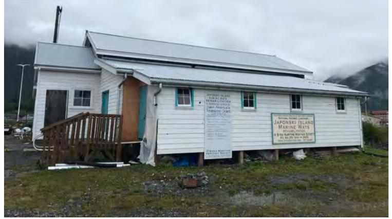
Top left: the NW side of the building, with work under way to repair original walls, and showing the accessible entry addition exterior. Plans call for a roofed deck on the right of the addition, with an accessible ramp and stairs to it.
