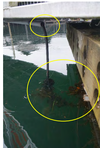
Photograph 21: Cable weighted by encrusted marine life and subject to chafing.
