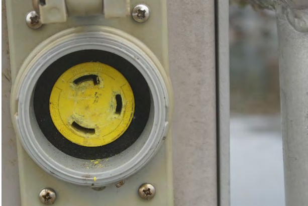
Photograph 22: Worn receptacle.
