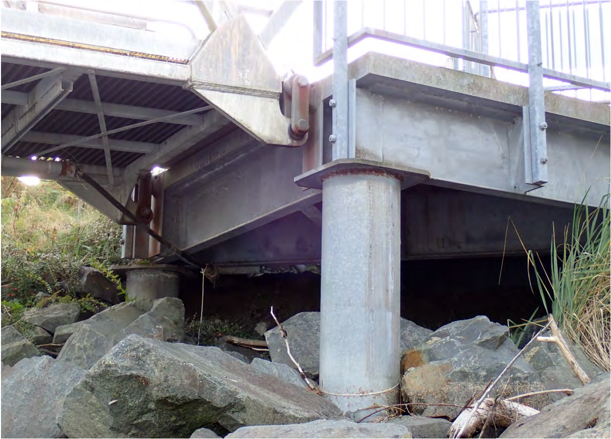
Photograph 15: View of the North Gangway abutment and connection hardware.
