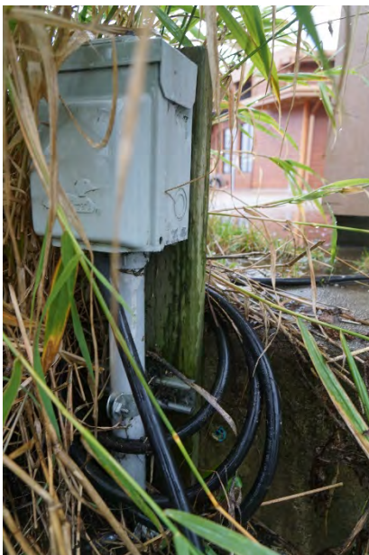
Photograph 24: Receptacle feeding outbuilding.
