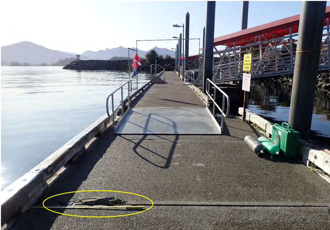
Photograph 1: View of the Lightering Float looking south with spall in the foreground.
