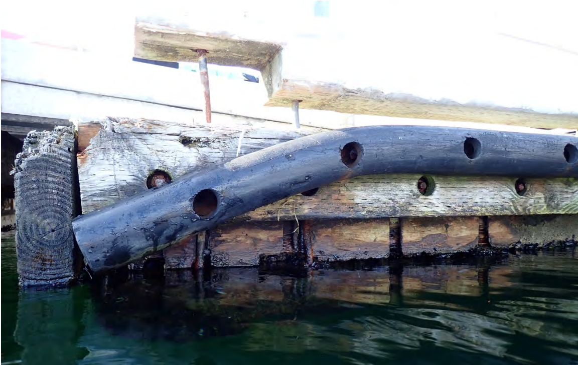
Photograph 7: View of the detached rubber 'D' fender at the southeast corner of Float 7.
