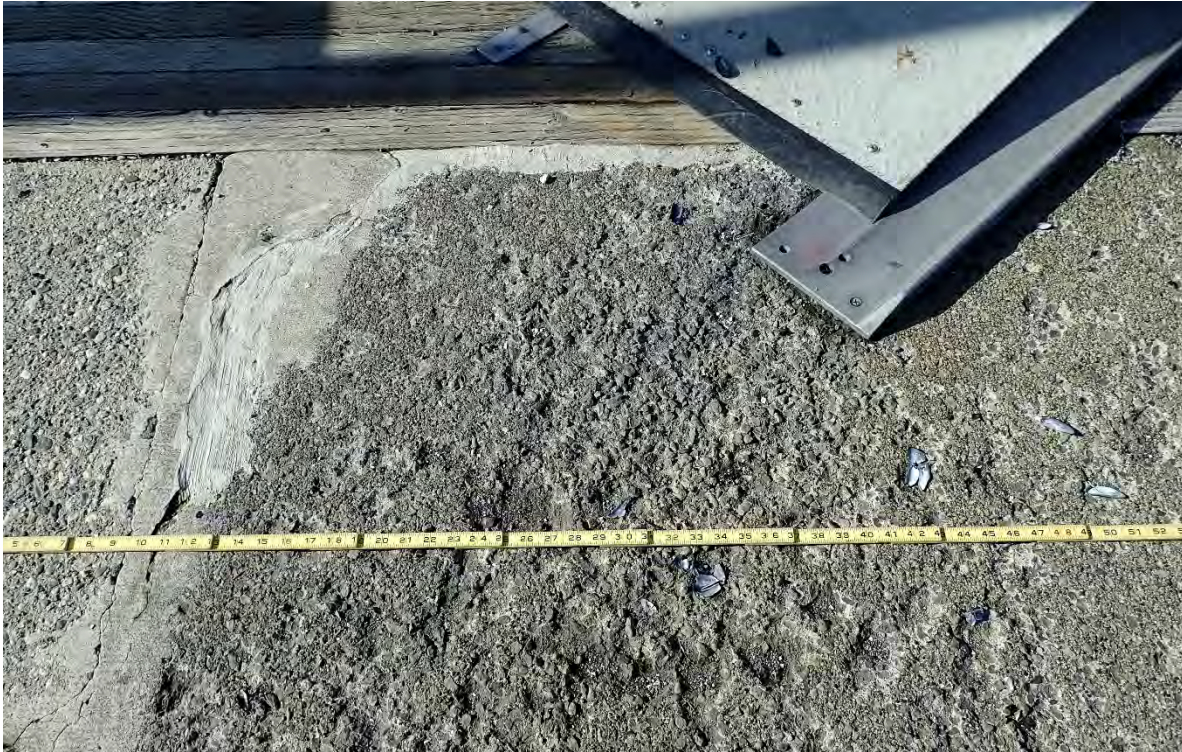
Photograph 3: View of scaling on topside of north gangway float.
