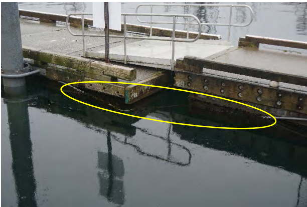
Photograph 16: Unfastened conduit.
