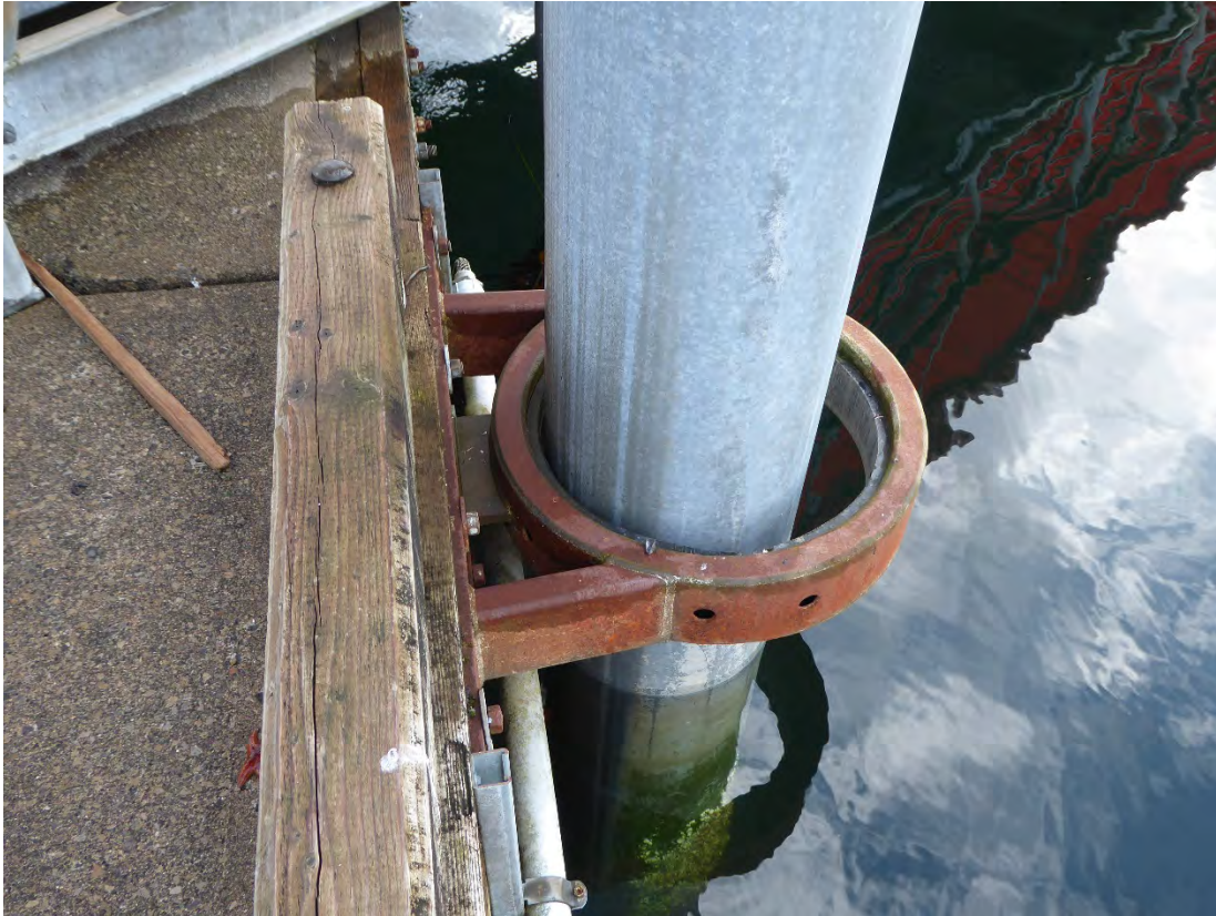
Photograph 13: Moderate corrosion at pile guide.
