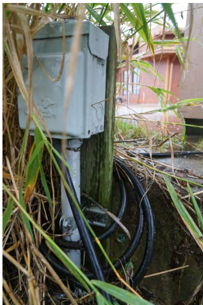
Photograph 24: Receptacle feeding outbuilding.
