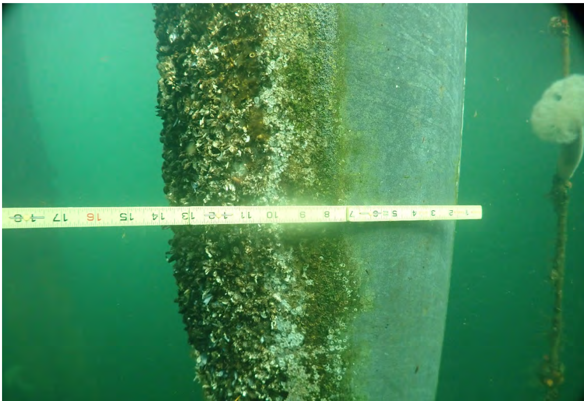
Photograph 10: View of typical galvanized steel pile condition below water.
