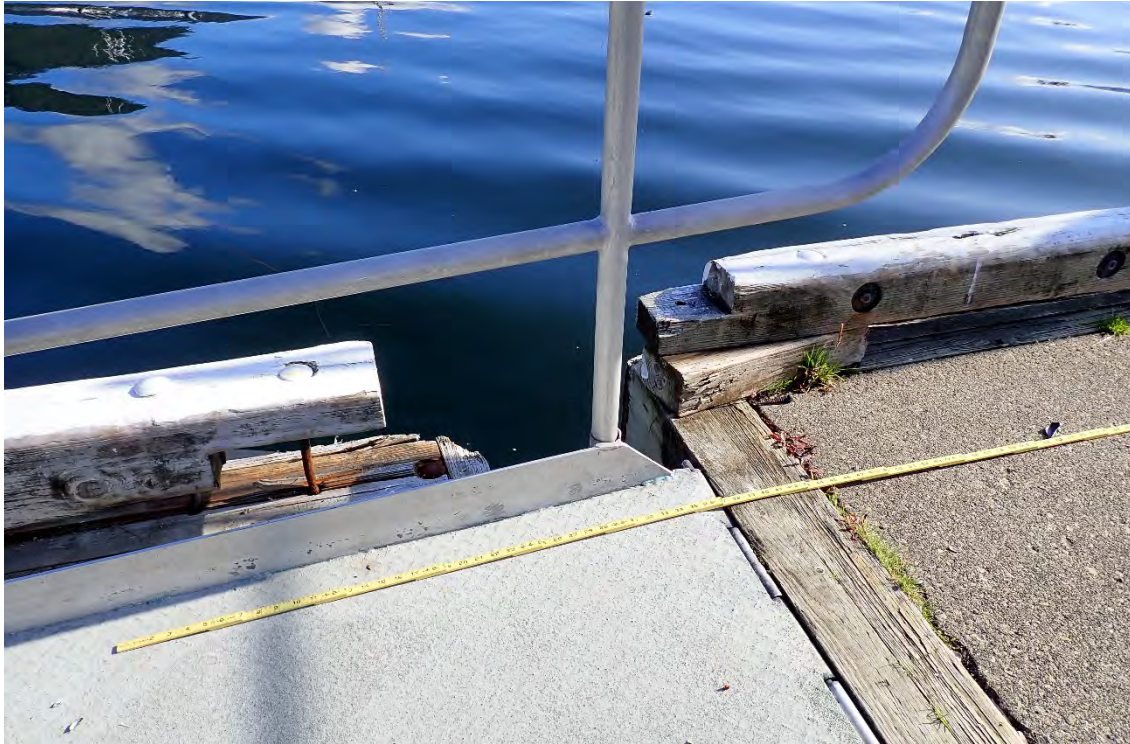
Photograph 5: View of the missing timber chock at southeast corner of Float 7.
