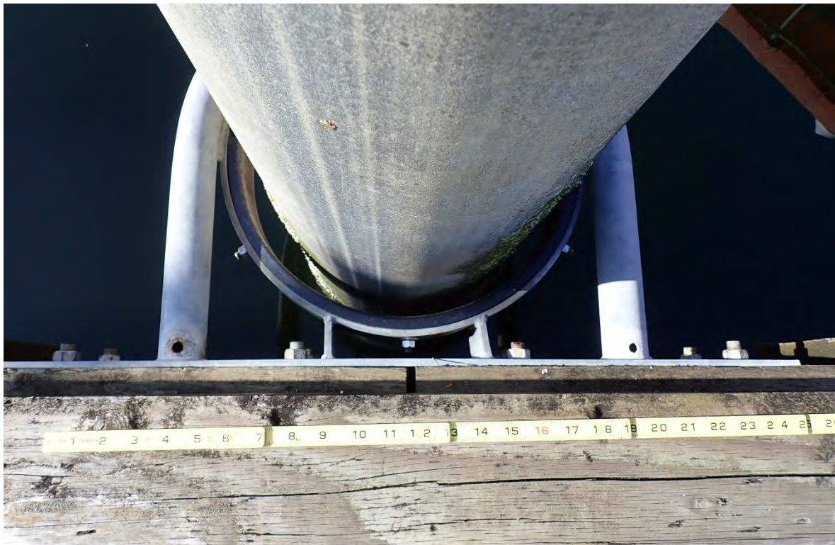
Photograph 12: View of pile guide installed upside down with weep holes on top surface.
