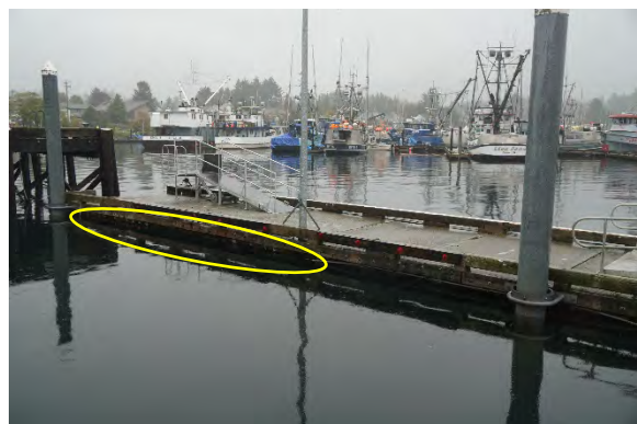
Photograph 17: Unfastened conduit.
