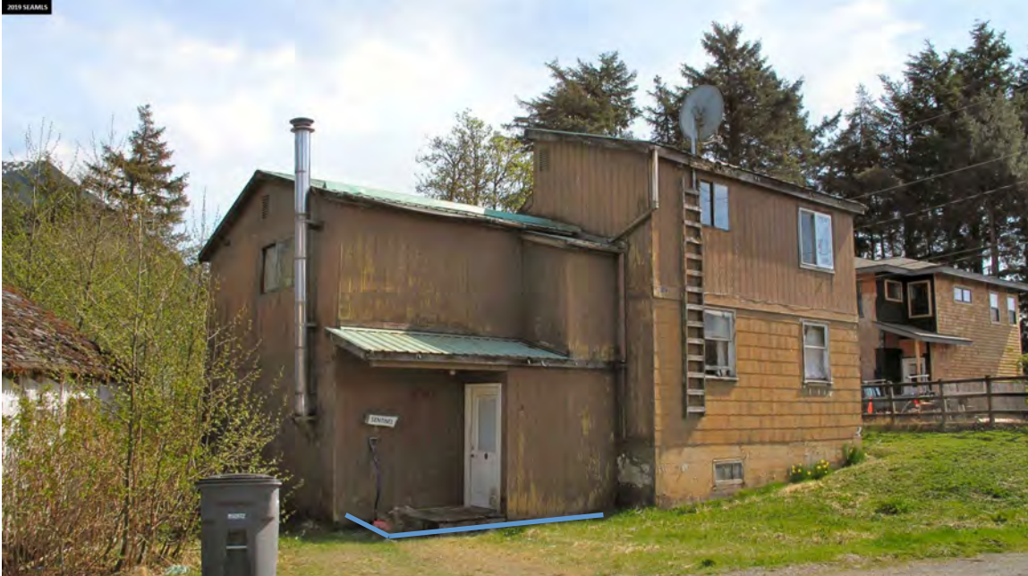
Figure 4. A foundation would run along the small porch, following the blue line. The current porch overhang is the footprint of this. The corner of the overhang is currently about 10 feet from the property line.
