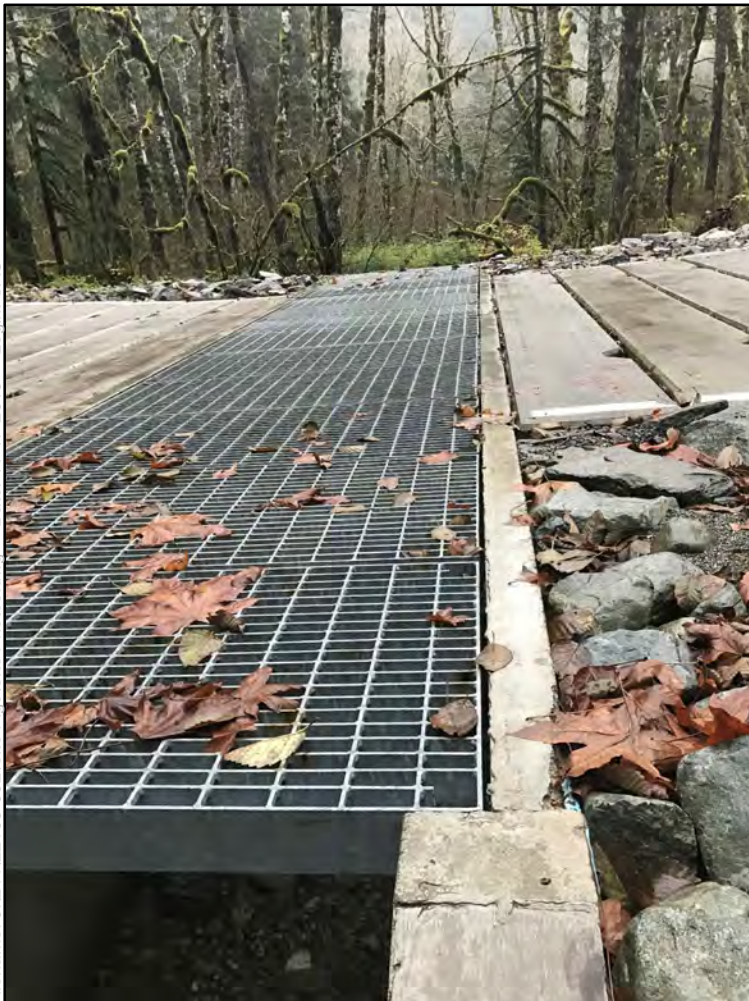
Photograph 22. Vented ford looking downstream through box culvert. Note articulated concrete mat and riprap erosion protection.
