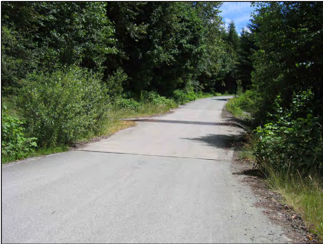
Photograph 18. Vented ford with steel grate cover over box culvert. Note concrete armor for flood flow.
