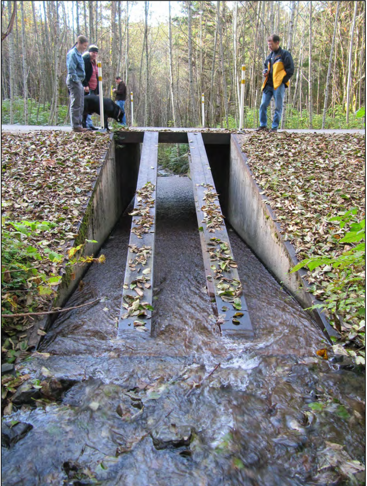
Photograph 21. Vented ford looking downstream through box culvert.
