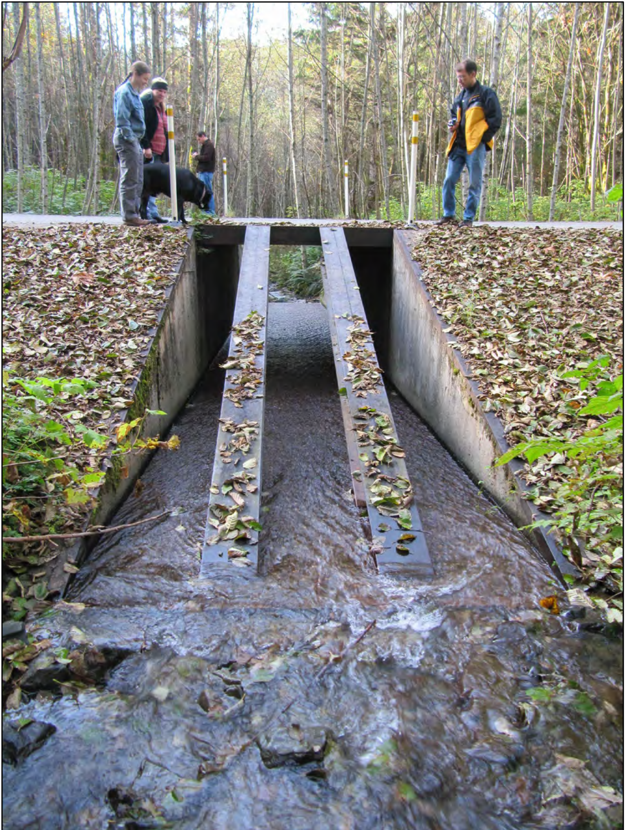
Photograph 21. Vented ford looking downstream through box culvert.
