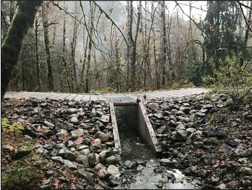
Photograph 22. Vented ford looking downstream through box culvert. Note articulated concrete mat and riprap erosion protection.
