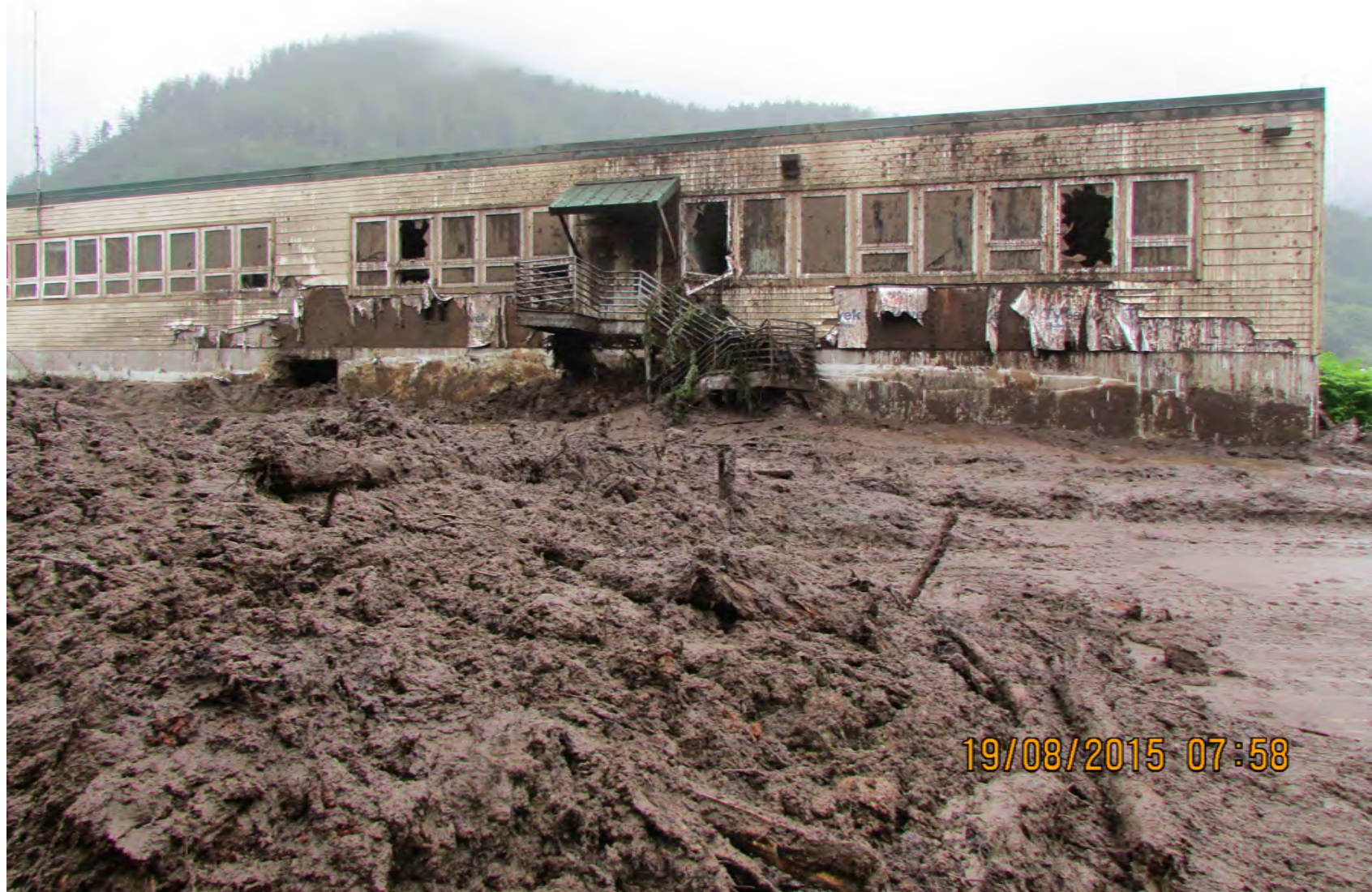
Photograph 3. Damage to Administration Building from Sawmill Creek Road debris flow. Photograph provided by CBS
