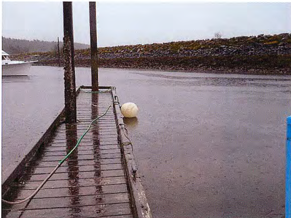
Rotting timber piles, worn bullrail and decking and loss of free-board on a typical Crescent Harbor finger float
