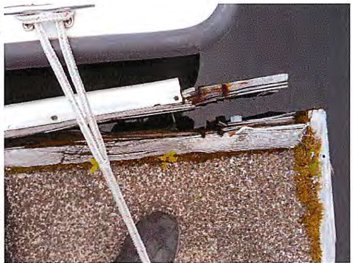
Damaged glulam
