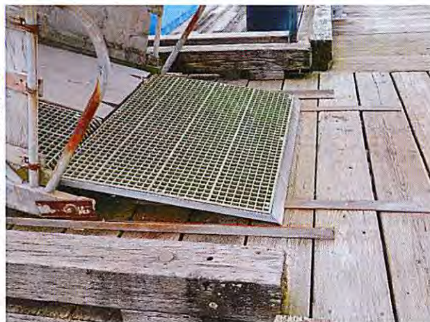
Trip hazard at gangway transition plate
