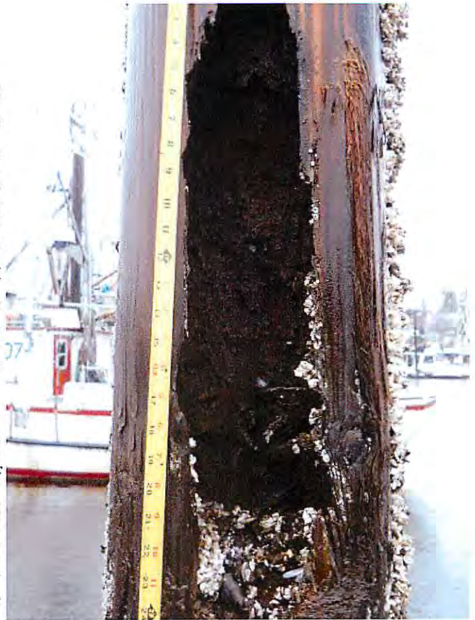
Extreme rot exhibited in timber piling. CBS has been methodically replacing timber piling as funding allows.
