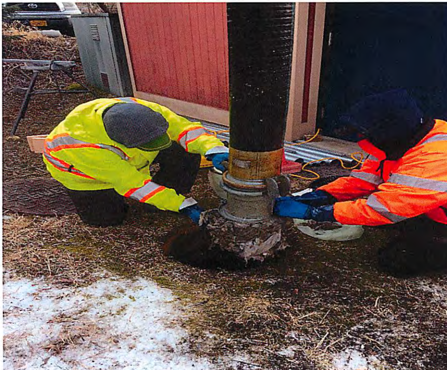
Removing wipes and such that have accumulated on the strainer of the bypass pump
