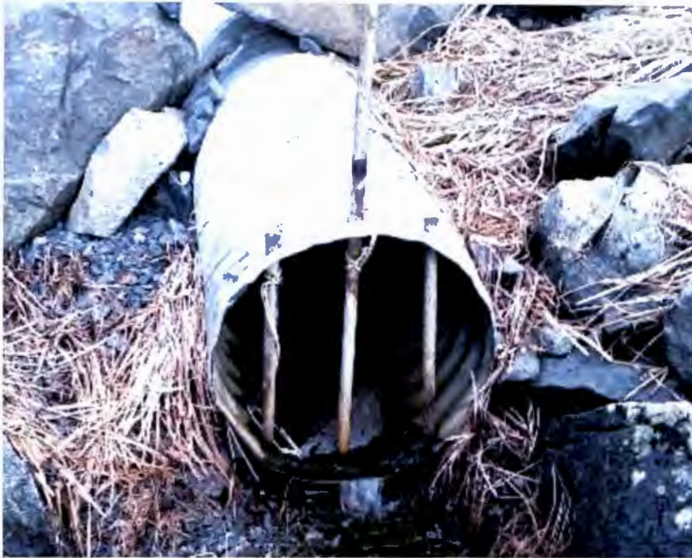
Outlet of 18" CMP on Lot #213 Showing Metal Bar Grating
