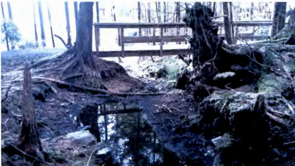
Looking Downstream at Sediment Accumulated above Manmade Dam. Dam is located at End of Pooled Water.
