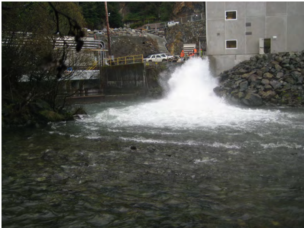
Figure 4: Penstock Drain Testing
