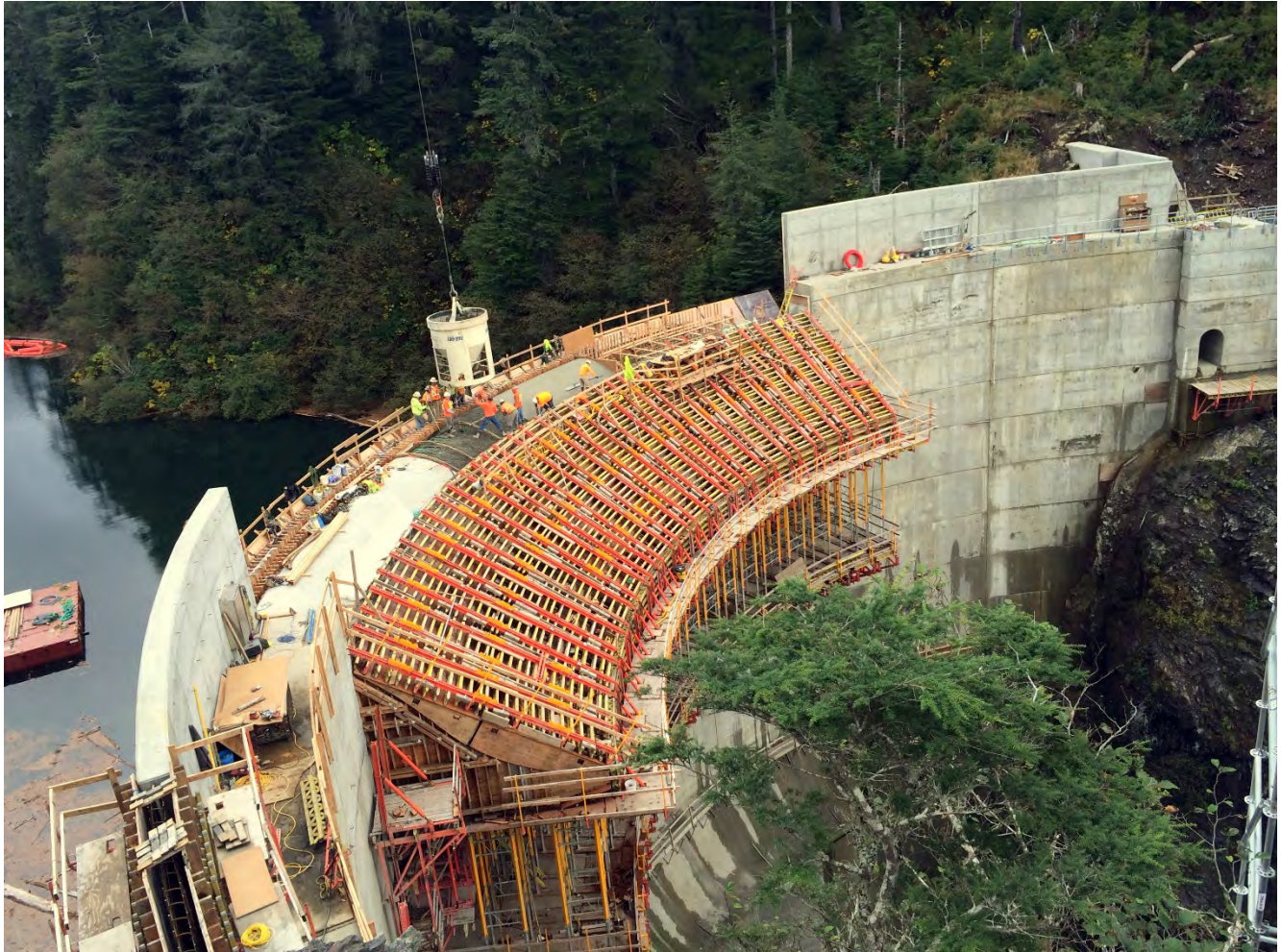
Figure 1. Dam and Left Abutment Area, Barnard crews completed 8 major concrete placements on the dam, including M1 crest slab, M3/425, M4/417, and 425, M5/417, Cutoff wall to El 440, M6 parapet wall and M7 parapet wall.
