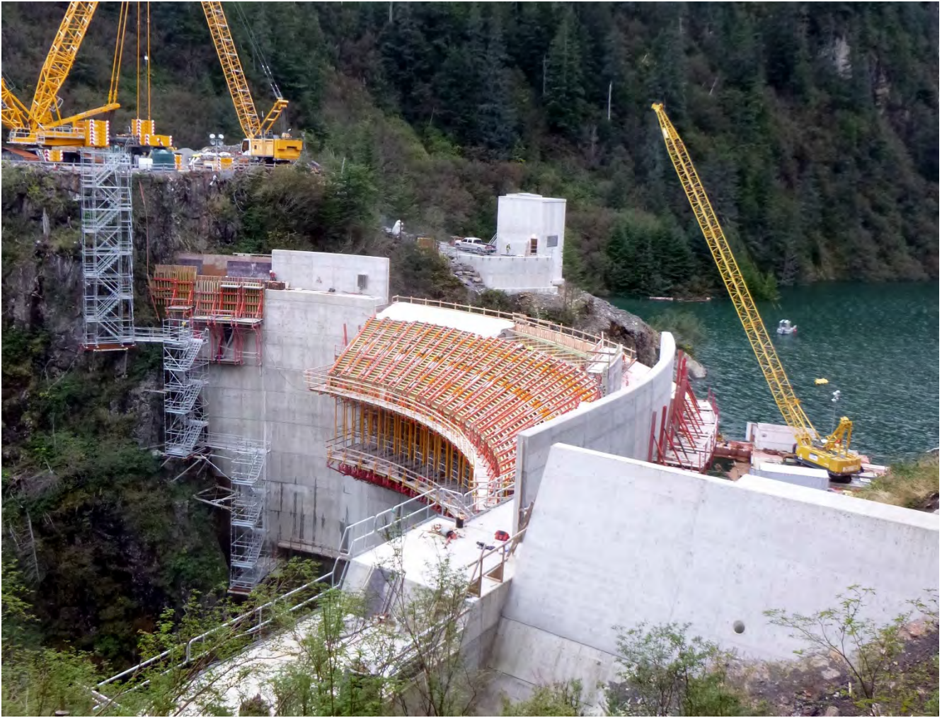
Figure 2. Intake Portal and Right Abutment, The concrete tunnel plug was completed in the existing intake tunnel. Tunnel and penstock were closed up in preparation for filling.
