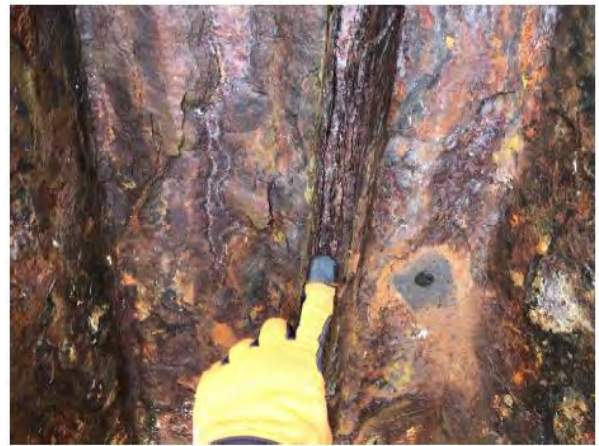
Figure 4- Sheet Pile Corrosion in Splash Zone, July 2021
