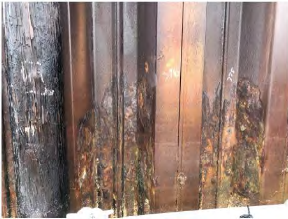
Figure 3- Sheet Pile Corrosion in Splash Zone, July 2021
