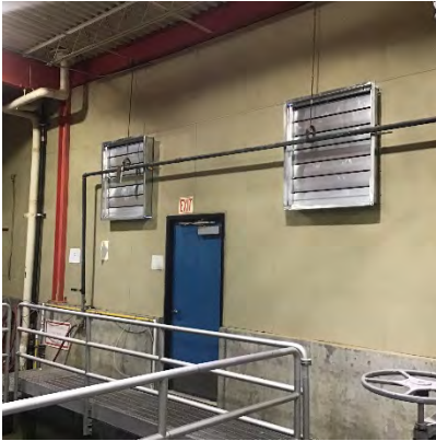
New louvers installed
