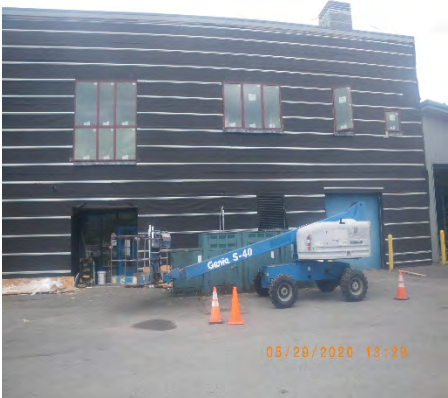
New windows installed
