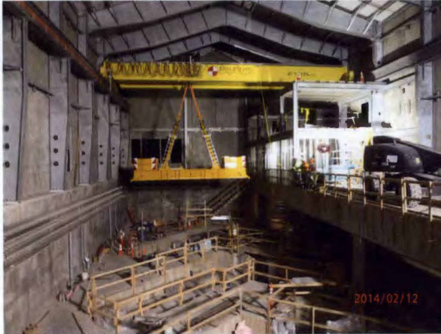
Figure 2: Bridge Crane Load Testing
