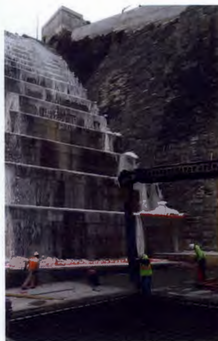
A crew places concrete in the plunge pool.
