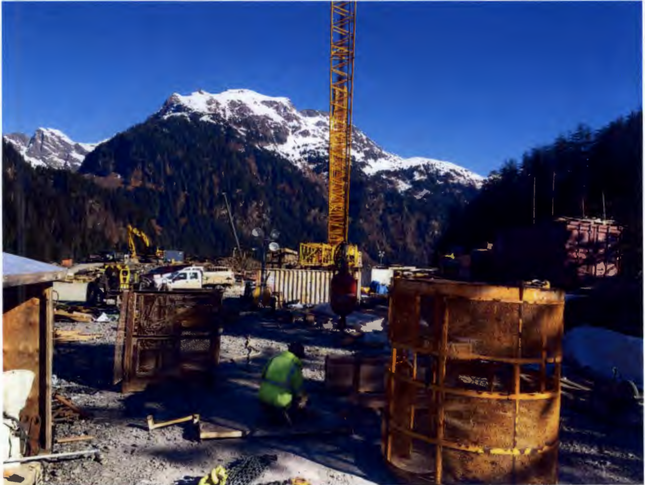
Figure 5. Dam Staging area, no change this month.
