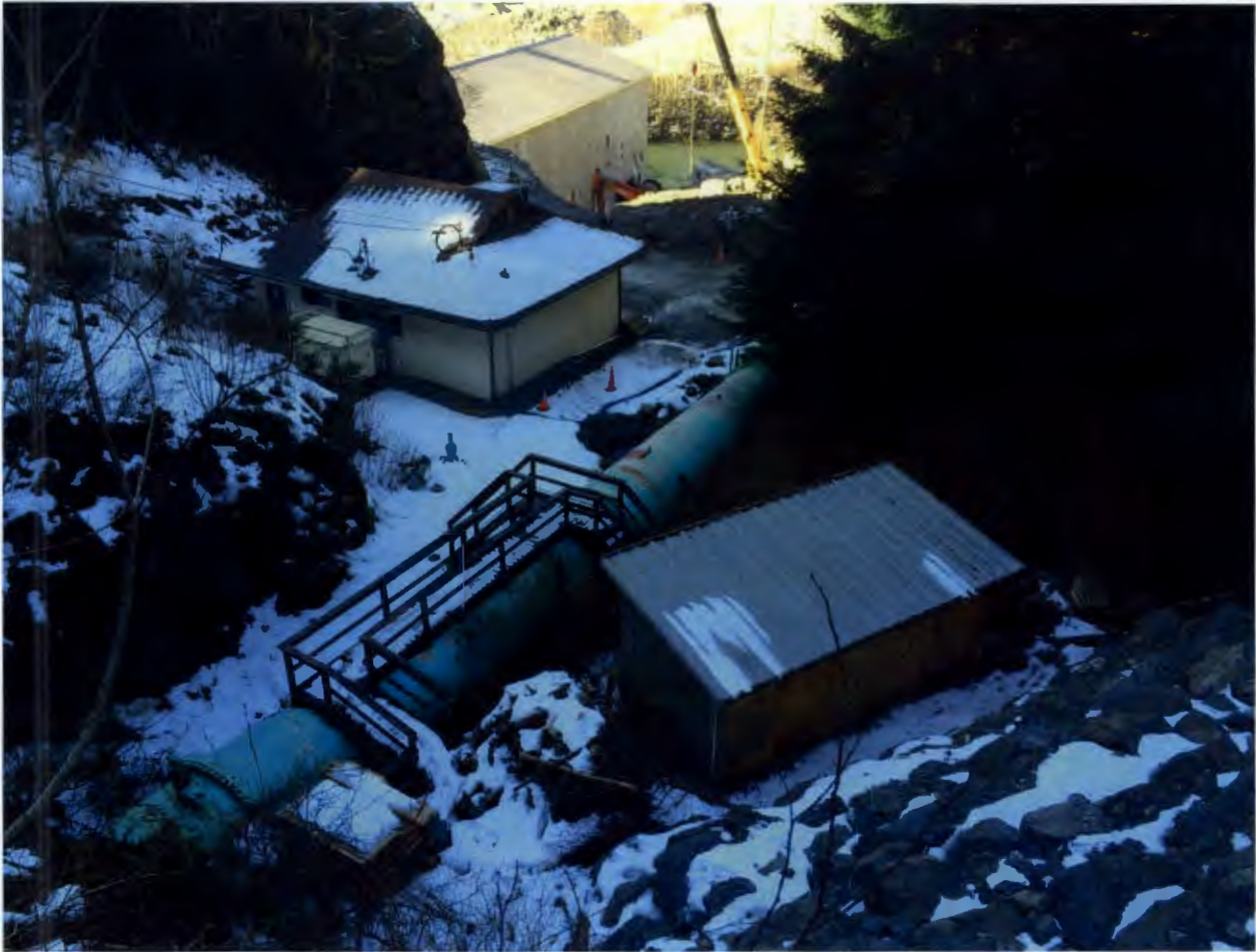
Figure 6. Lower Portal Area, Excavation began for upper penstock sections
