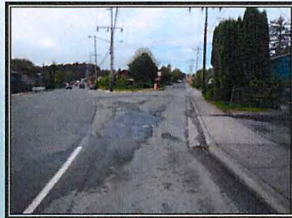
Existing DeGroff/SMC intersection
