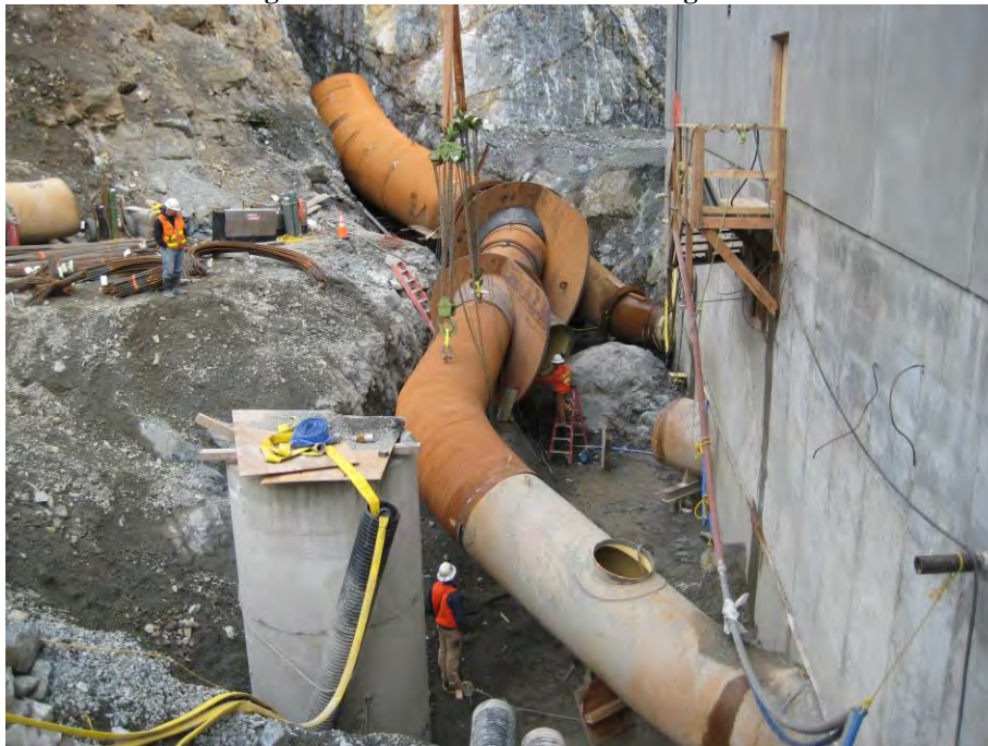
Figure 4: Penstock Installation
