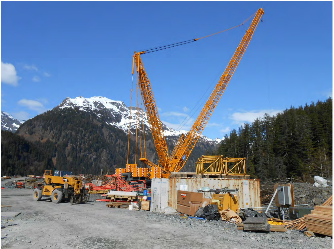
Figure 5. Dam Staging area, no change this month.
