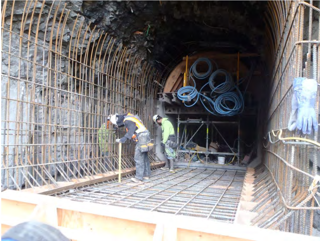
Figure 3: Gate Chamber Reinforcing Steel
