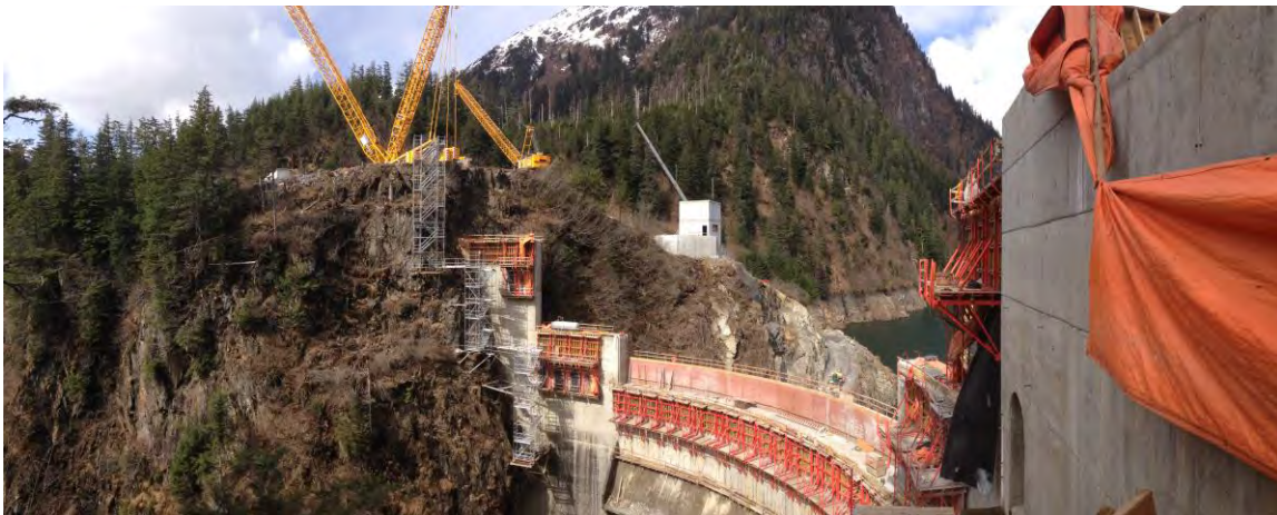
Figure 1: Dam Raise From Left Abutment
