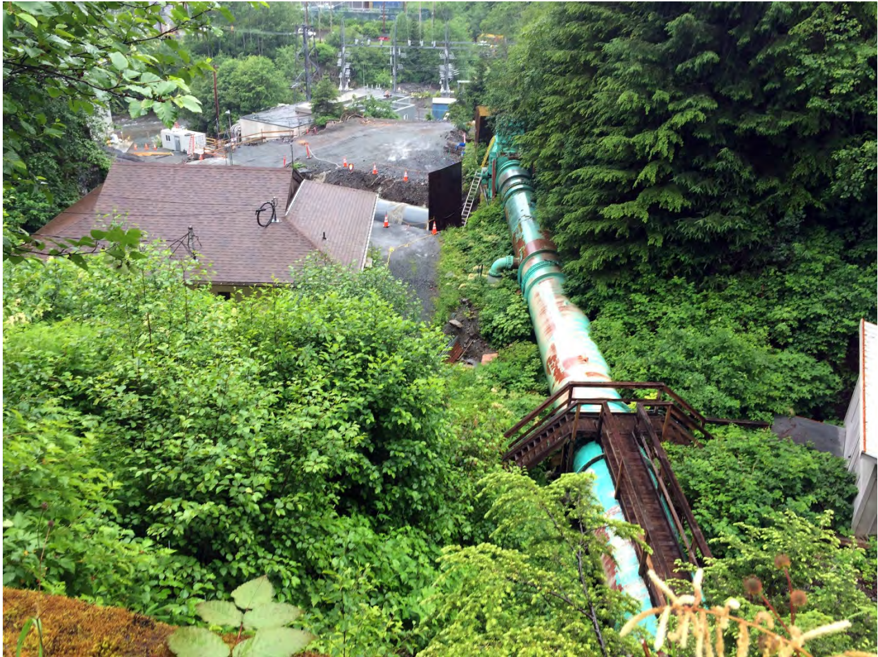
Figure 6. Lower Portal Area, No change this month.
