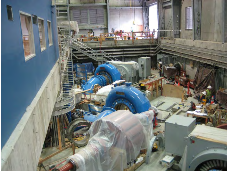
Figure 1: Powerhouse Turbine Floor
