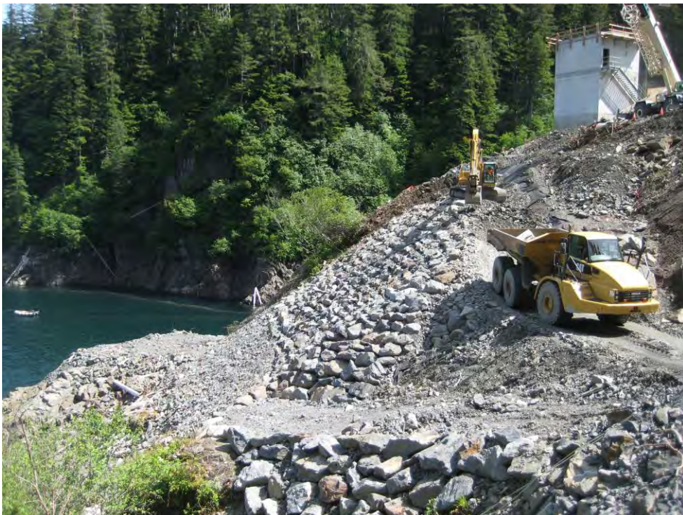
Figure 6: Access Road Slope Protection
