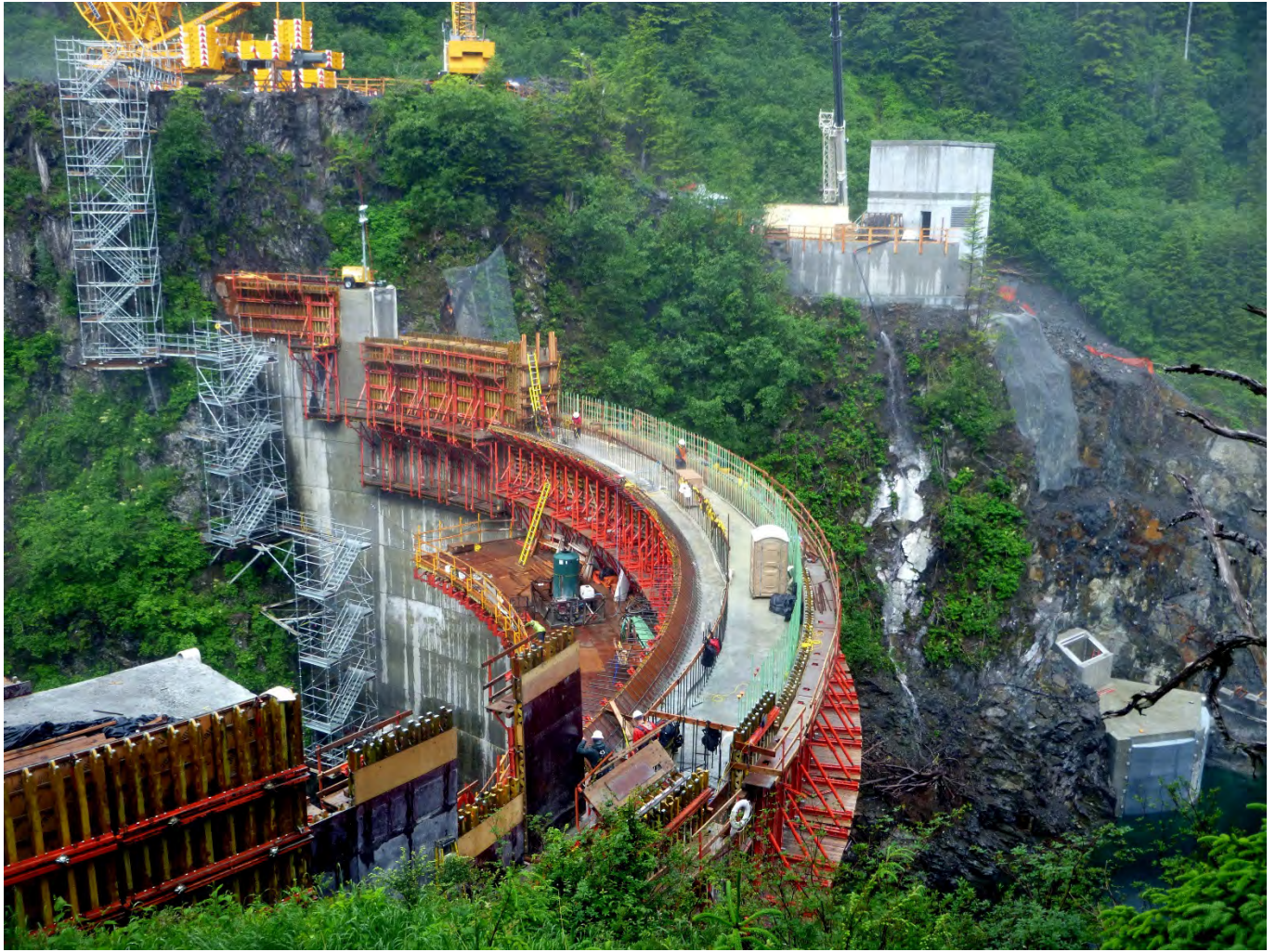
Figure 3. Intake Portal and Right Abutment, Barnard completed the new tunnel intake structure on time, Project Milestone No. 4. The new intake structure is now 50% submerged.
