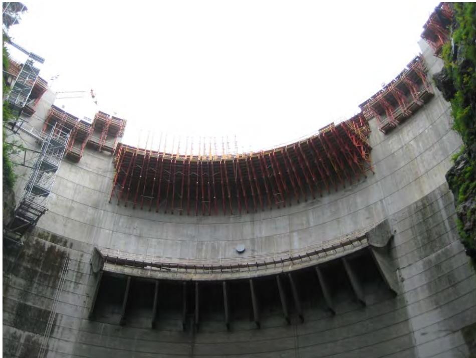
Figure 4: Dam Raise View from Plunge Pool
