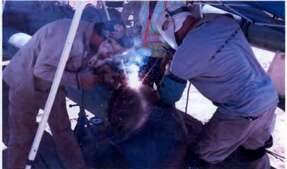
Welders weld a 16-inch tie-in assembly.
