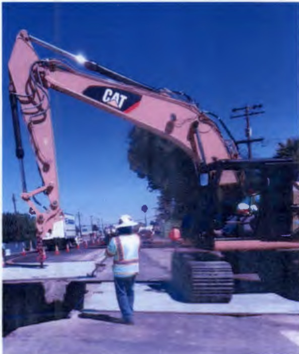
Excavation at the West Sacramento project.
