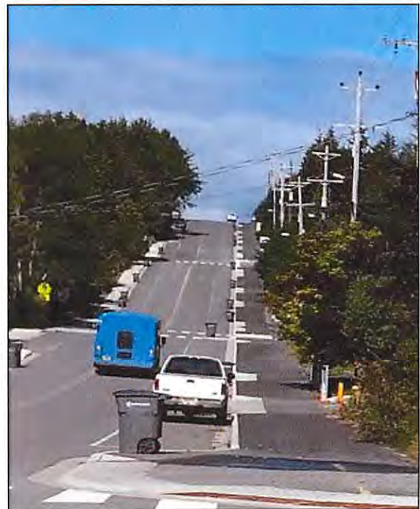
Partial-width concrete driveway cuts are shown in the asphalt-paved Edgcumbe Drive multi-use path. Public Works recommends partial-width cuts and asphalt surfacing if the Assembly chooses ADOT’s Option 2 alignment.
