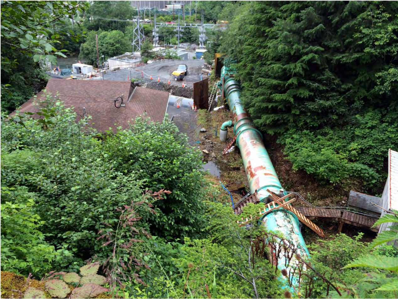
Figure 6. Lower Portal Area, Barnard prepared the penstock for generation outage work.
