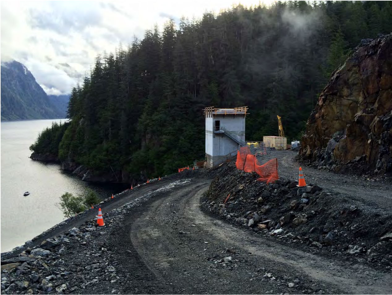
Figure 4. Gate House Location, Barnard completed the reservoir access road.
