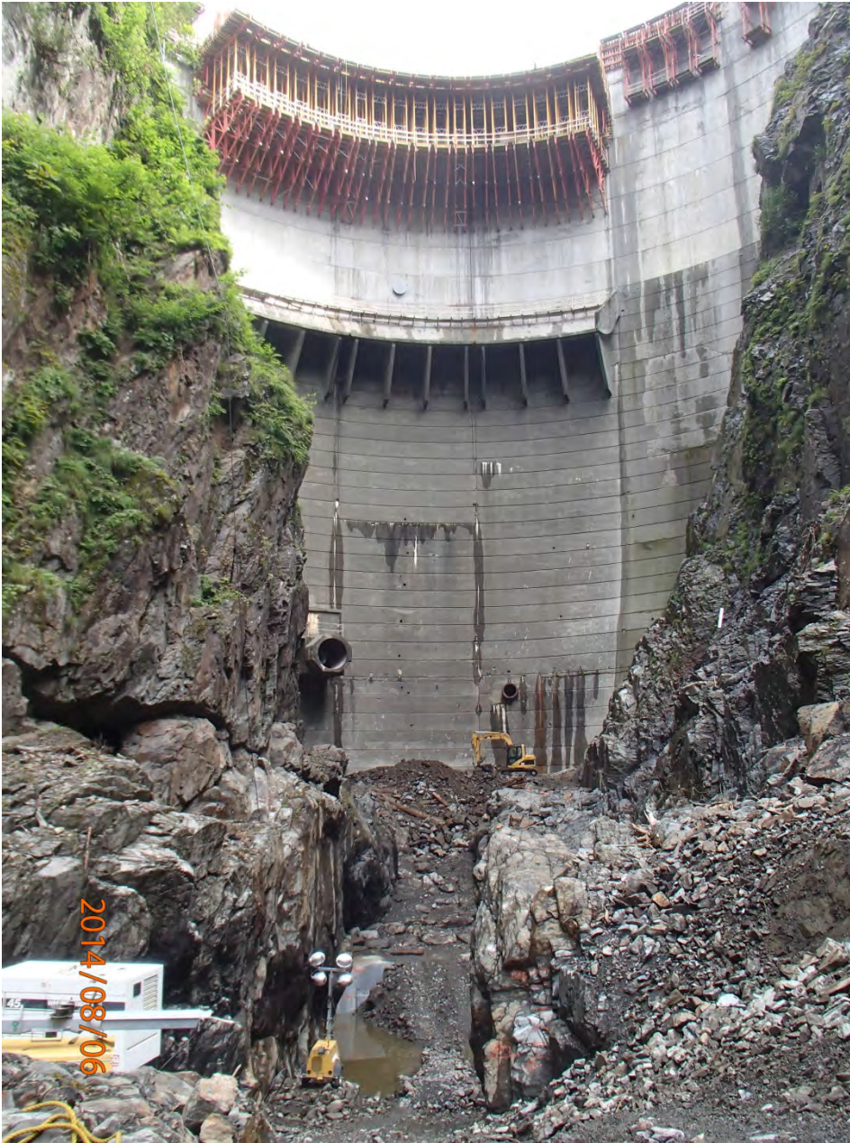
Figure 2. Drainage Tunnel and Scour Wall, Crux completed the scour wall.
