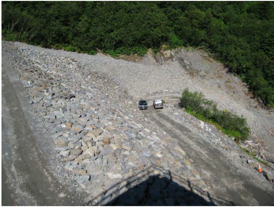
Figure 5: Completed Reservoir Access Road
