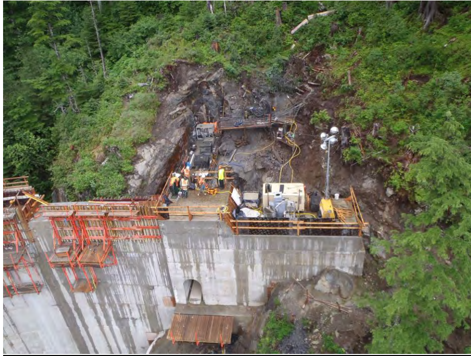
Figure 2: Left Abutment Curtain Grouting
