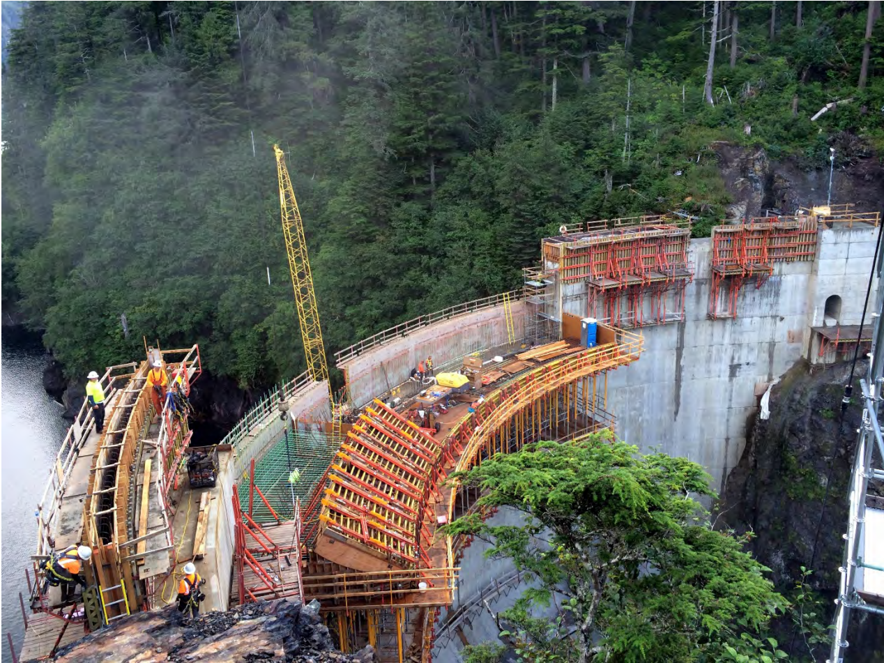
Figure 1. Dam and Left Abutment Area, Barnard showed good progress on the dam construction completing 2 block placements . TO DATE – 53 of 53 blocks placed on the Dam Raise. In June Barnard started work on the spillway section of the dam, which is the most complicated formwork for the dam raise. Eight of 9 placements completed on the Left Abutment and Cutoff Wall. Crux completed all curtain grout holes on the left abutment.
