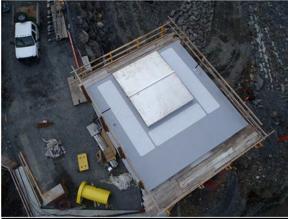
Figure 4: Gate House Roof and Hatch
