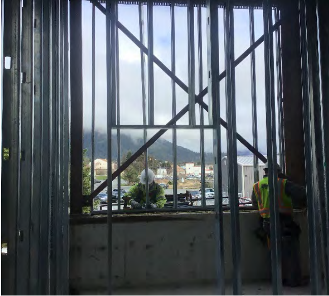
New interior framing
