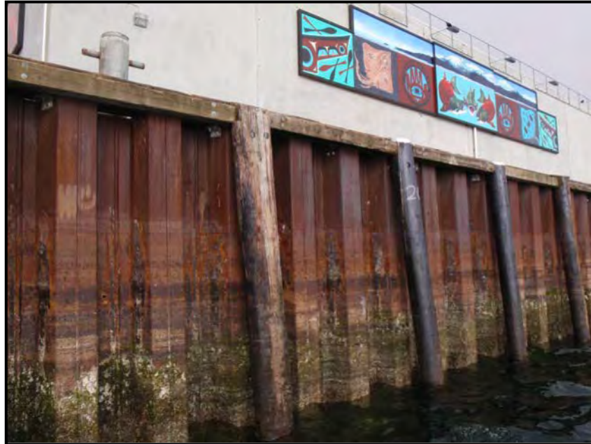
Figure 1 – Segment of Sheetpile Bulkhead Face – July 2011
