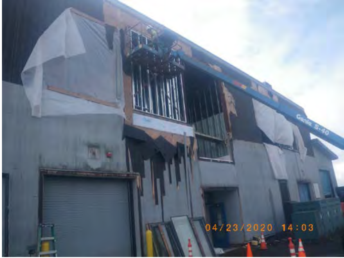
Exterior siding demo
