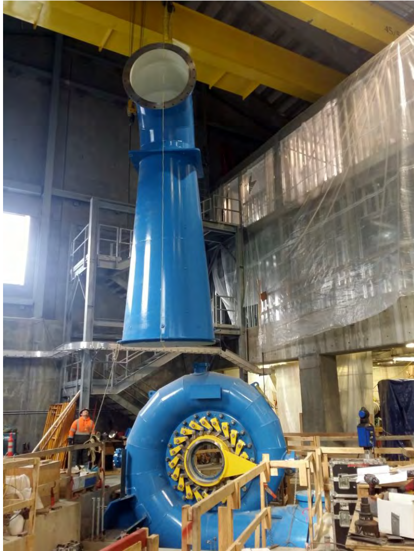
Figure 5: Unit #5 Draft Tube Installation
