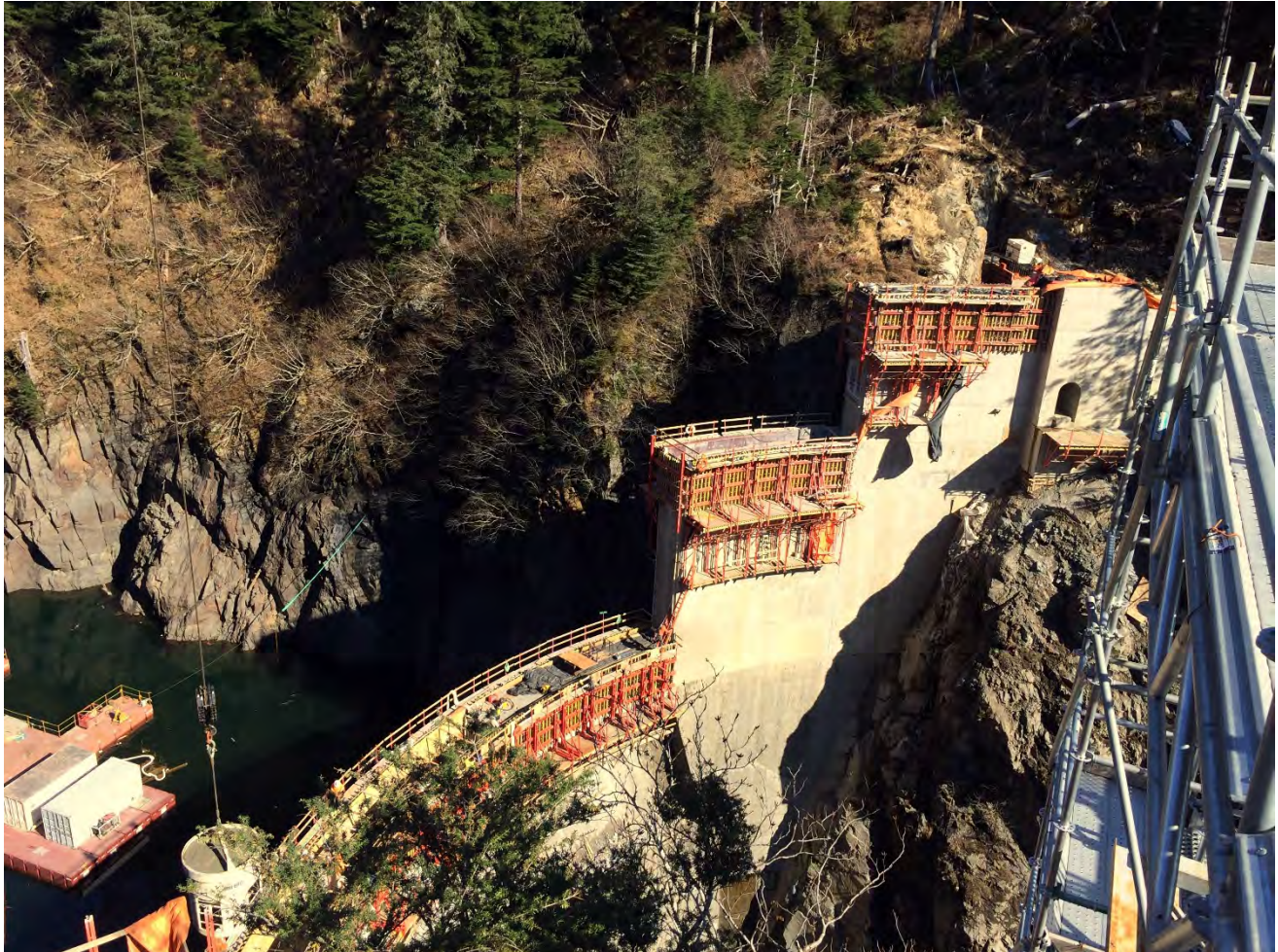
Figure 1. Dam and Left Abutment Area, Barnard made final concrete placement on dam keyway and began forming for dam raise blocks M3-M5 (in the old spillway).
