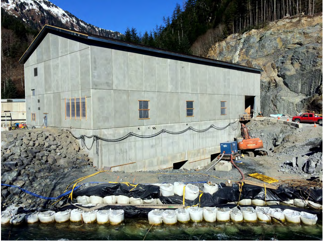
Figure 7. Powerhouse Site, Southeast Earthmovers began the powerhouse afterbay excavation.
