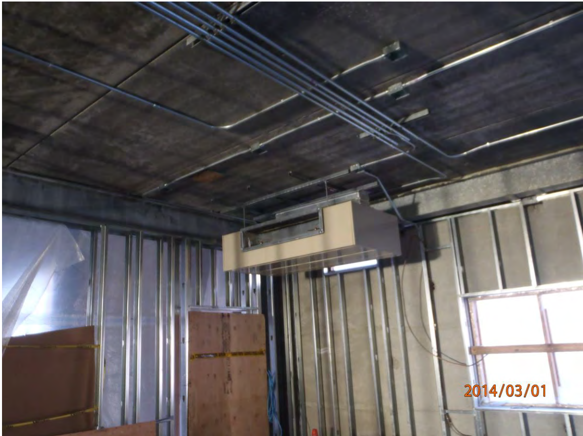
Figure 4: Powerhouse Interior Buildout
