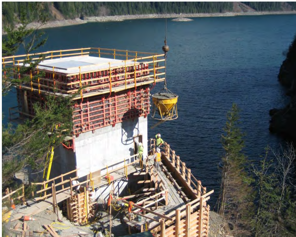
Figure 2: Gatehouse Retaining Wall Placement
