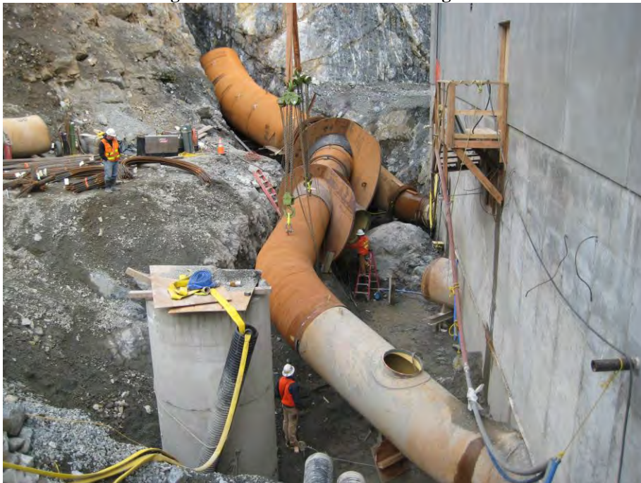
Figure 4: Penstock Installation
