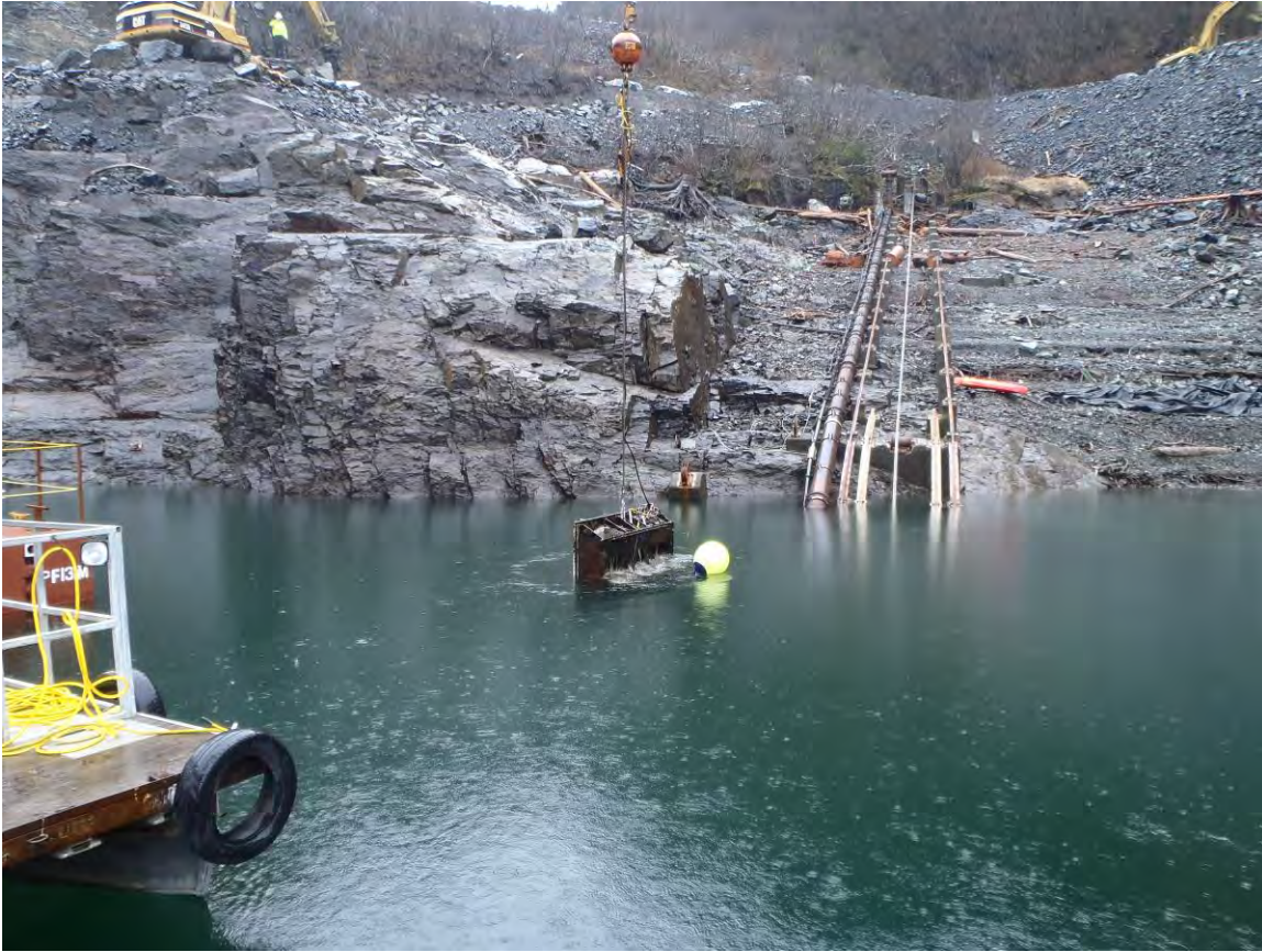
Figure 2: Removing Existing Bulkhead Gate
