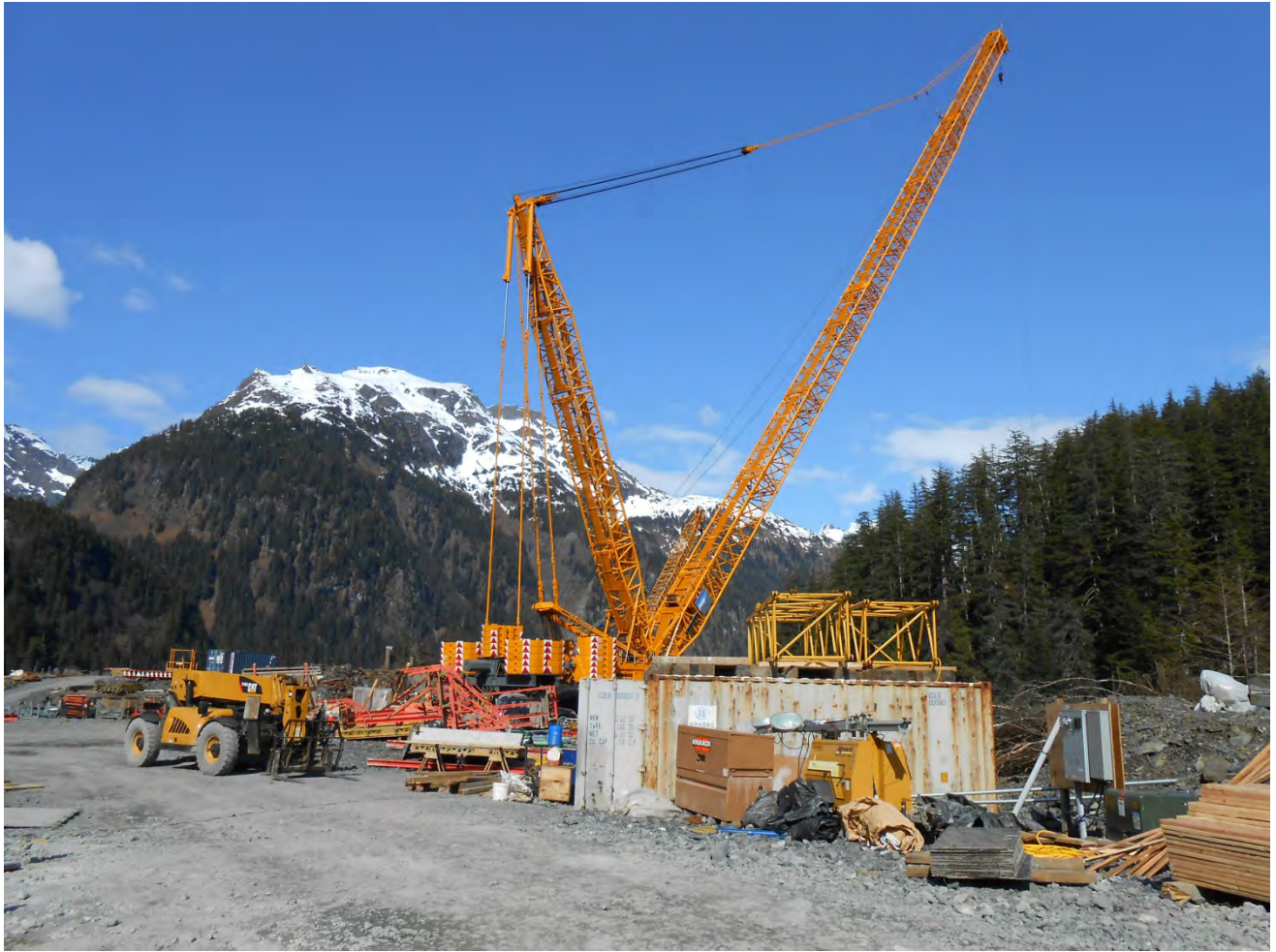
Figure 5. Dam Staging area, no change this month.
