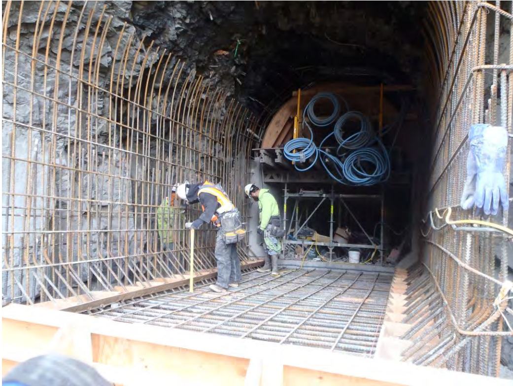
Figure 3: Gate Chamber Reinforcing Steel
