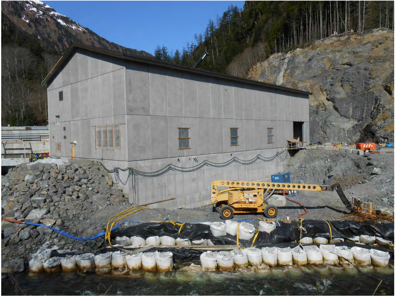
Figure 7. Powerhouse Site, no change this month.
