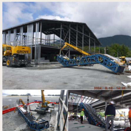
Airport escalator install
