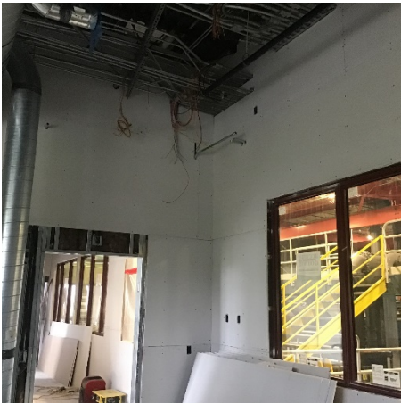
Sheetrock installation
