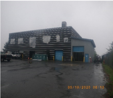
Hat channel and felt paper installed. Preparing for new windows.
