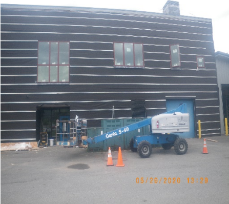
New windows installed
