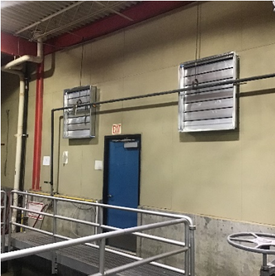
New louvers installed
