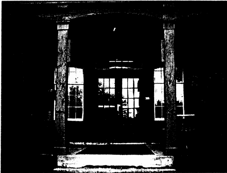
Porch detailing: wood columns with capital and base detail, low segmental arches, wood railing.
