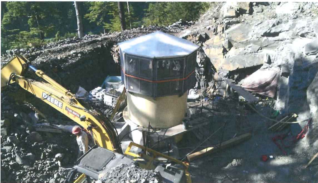
Figure 3: Surge Shaft Top Structure
