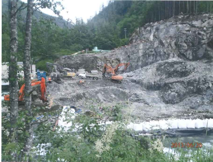
Figure 4: Powerhouse Excavation
