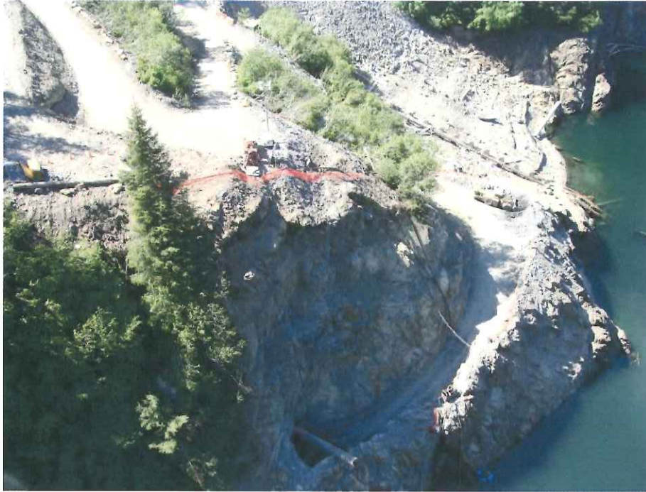
Figure 2: Aerial View of Intake Tunnel Portal
