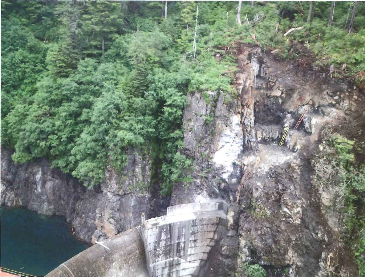
Figure 1. Dam and Left Abutment Area, Blue Lake Tunnelers completed the left abutment thrust block excavation. Work on the keyway began and the first concrete pour was completed on the dam.
