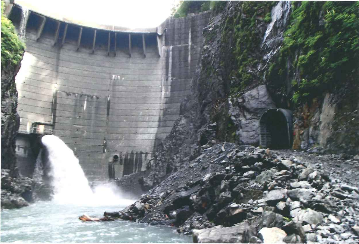
Figure 2. Drainage Tunnel and Scour Wall, the Howell Bunger valve was opened to 10% to control the rising lake level.
