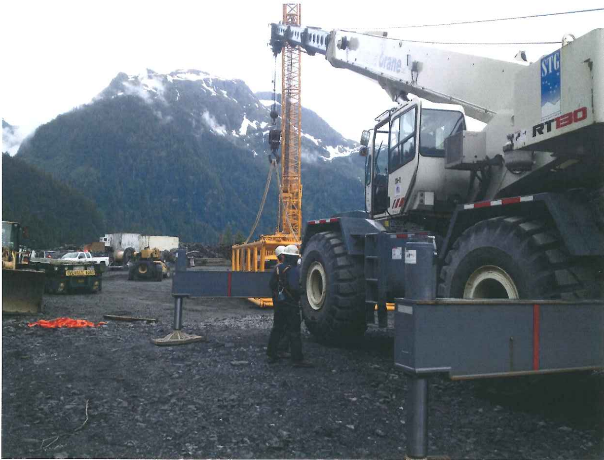
Figure 5. Dam Staging area, The 600 ton crane boom was disassembled to add an additional 40 feet of boom and a new counter weight carriage.
