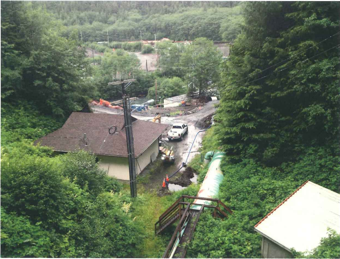
Figure 7. Lower Portal Area, No change this month.
