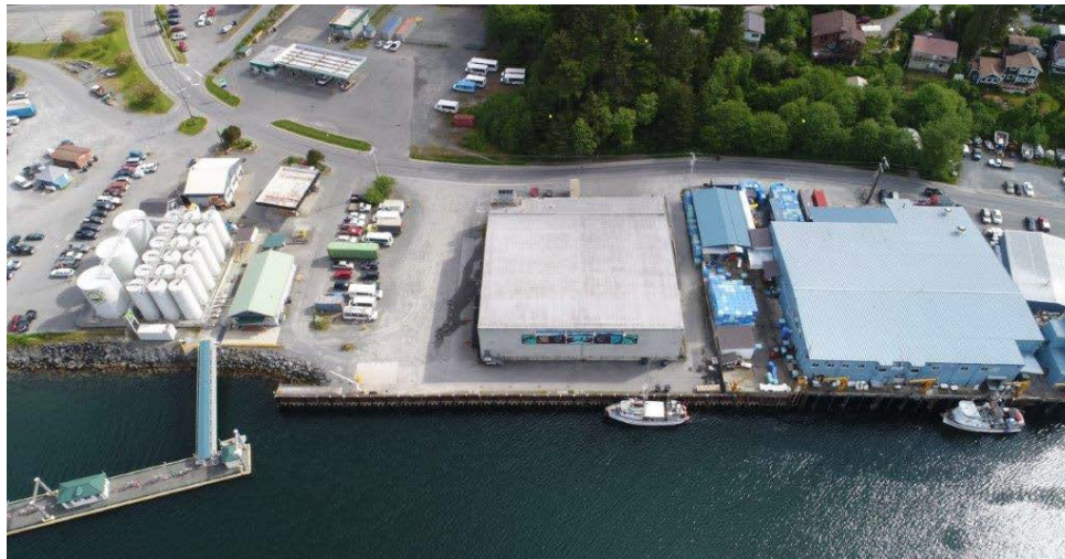
Figure 5 – Marine Service Center Cold Storage Facility and Adjacent Seafood Processing Plant
