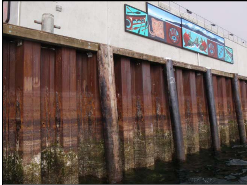
Figure 1 – Segment of Sheetpile Bulkhead Face – July 2011
