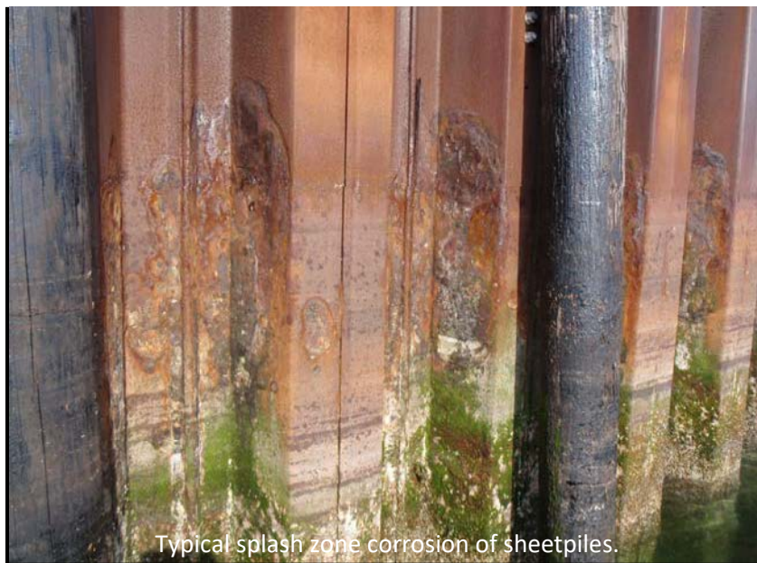
Figure 2 – Splash Zone Corrosion of Sheetpile – July 2011
