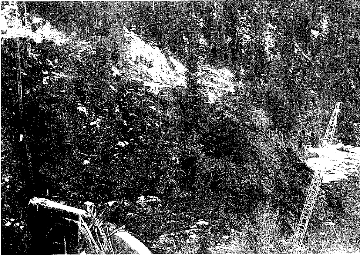
Figure 3. Intake Portal and Right Abutment, Excavation to the gate house and the intake access road has begun.
