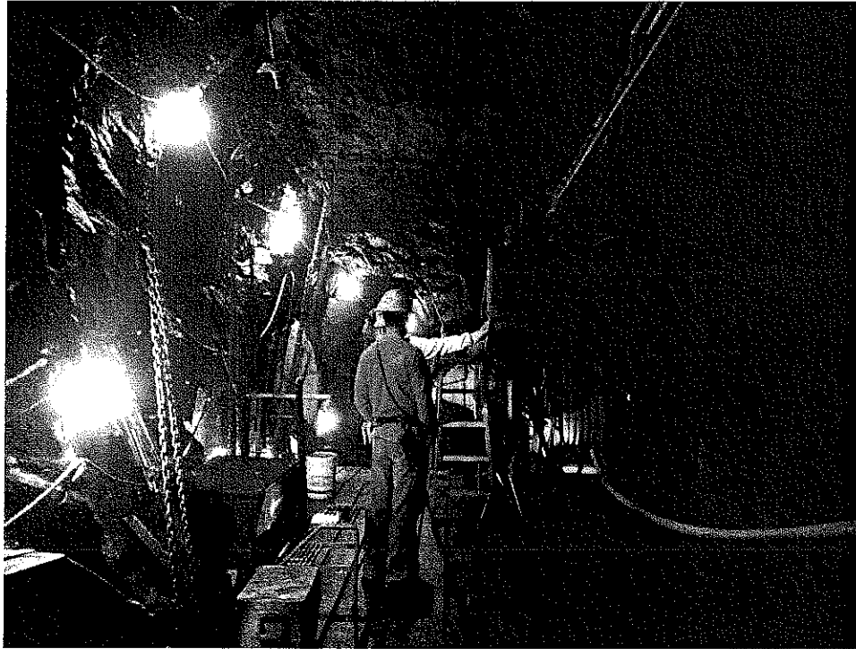
Figure 6: Alimak Raise Climber Platform at Surge Shaft
