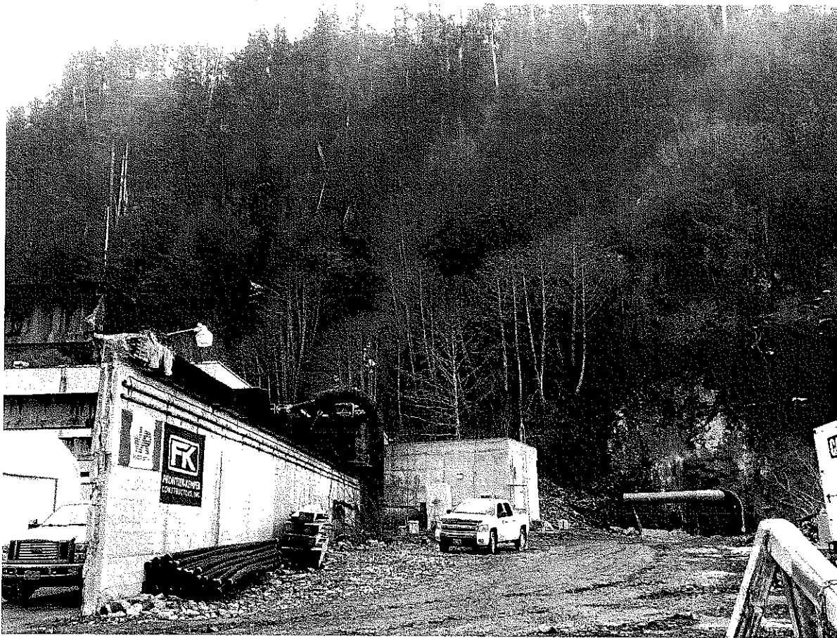
Figure 6. Surge Chamber, the 470' adit was completed in February and while it is unseen here, work on the raise of the surge shaft is ongoing.
