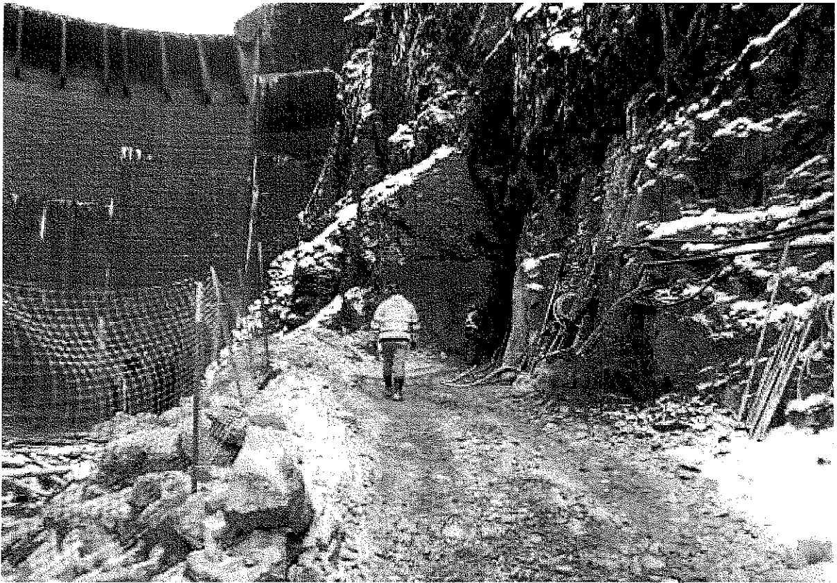
Figure 2. Drainage Tunnel and Scour Wall, Excavation of the drainage tunnel in the dam left abutment has begun.
