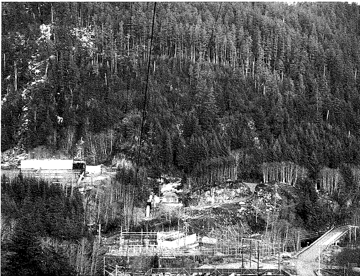
Figure 8. Lower Project Site, Clearing for the surge chamber top portal and continuing powerhouse excavation can be seen.
