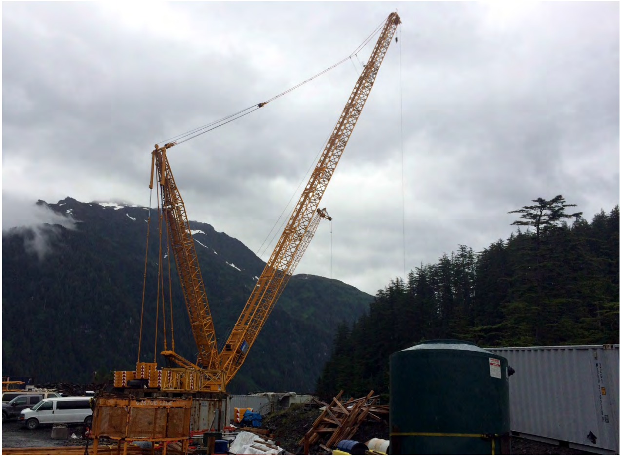
Figure 5. Dam Staging area, no change this month.
