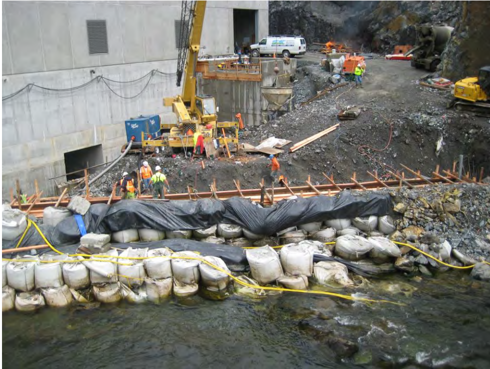
Figure 3: Afterbay Concrete Weir Placement
