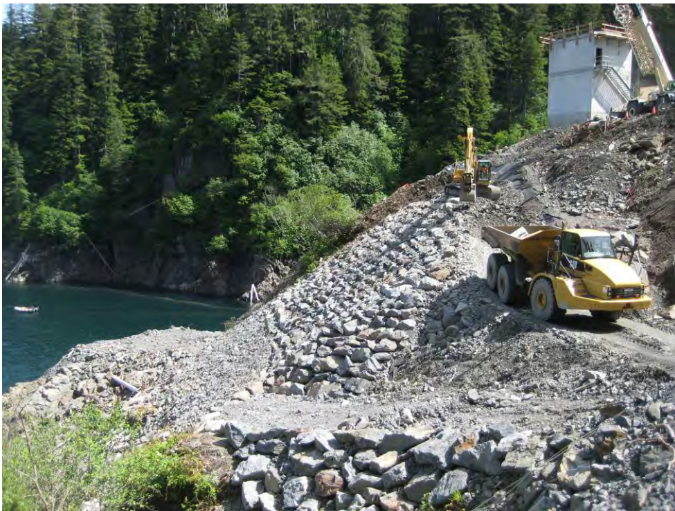
Figure 6: Access Road Slope Protection
