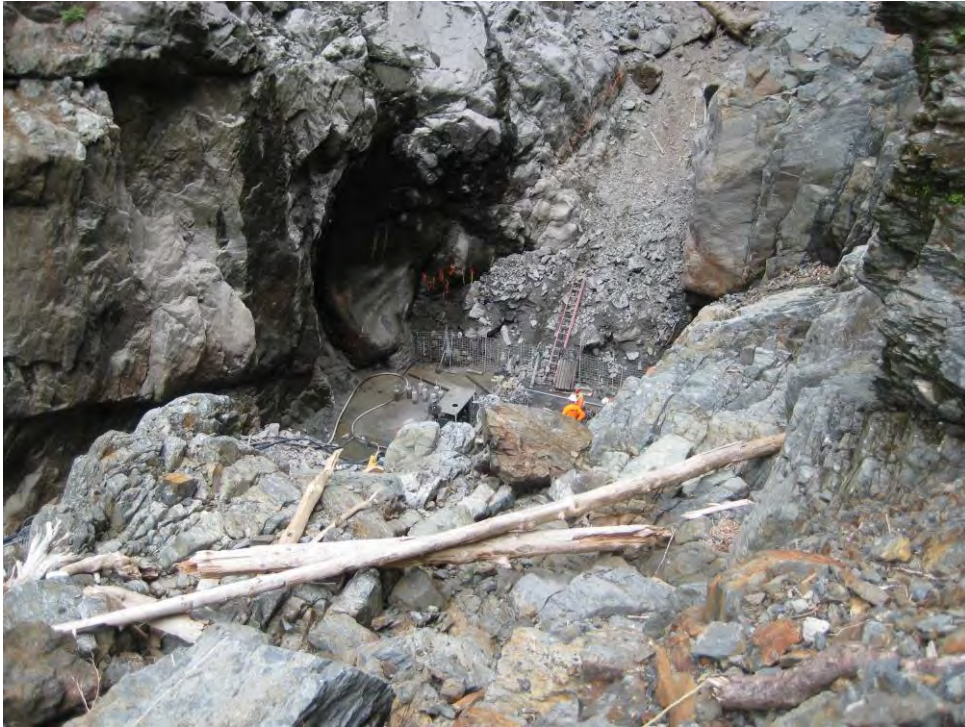
Figure 5: Micropile Installation in Plunge Pool
