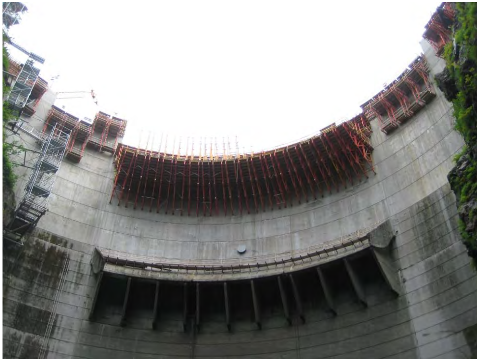
Figure 4: Dam Raise View from Plunge Pool
