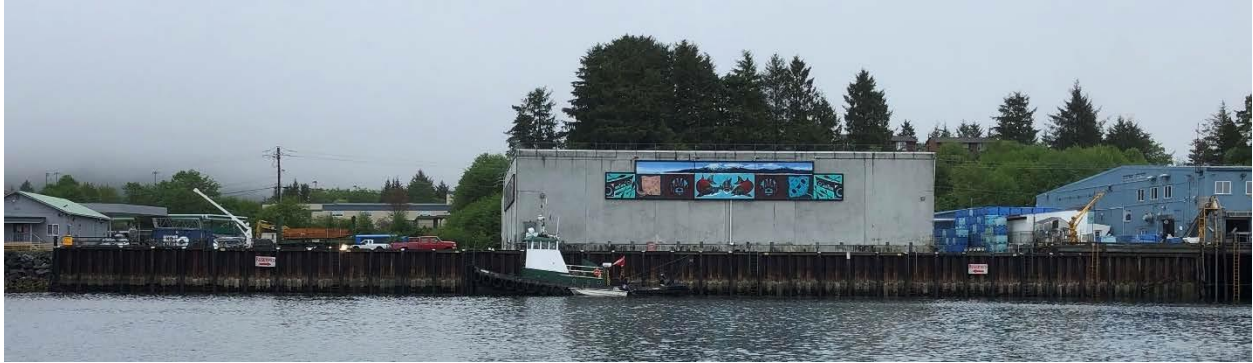
Marine Service Center Sheet Pile Wall and Crane
