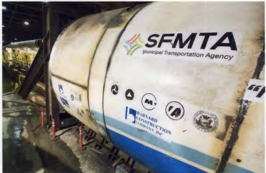
Crews prepare the Central T TBM, “Mom Chung,” for launch.
