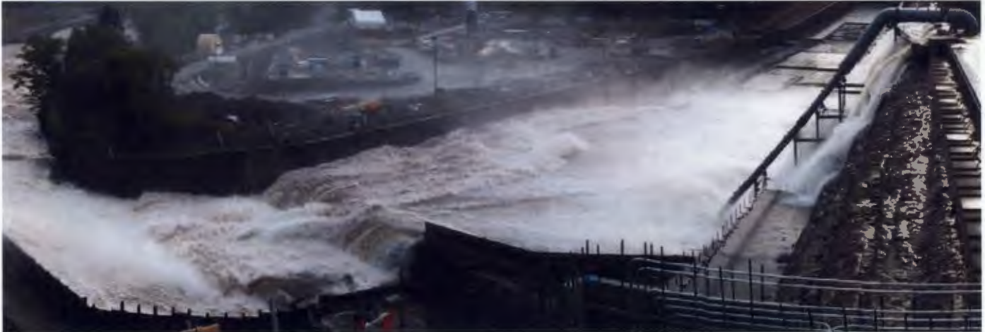
Spillway flows nearly exceeded the crest notch capacity of 8,000 cubic feet per second at Gilboa Dam in mid-June.
