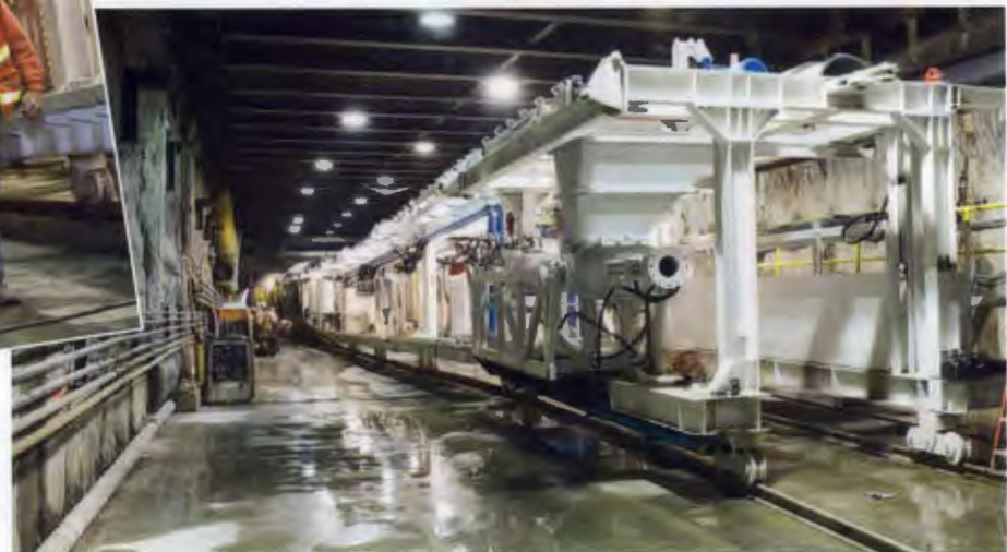
Above, Shift Superintendent Bill Kiehl (right) and crew plan the day's work. At right, a view of the TBM trailing gear during testing and commissioning.
