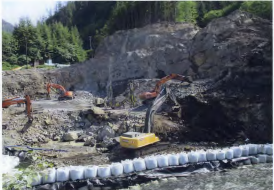
Above, powerhouse excavation is underway along Sawmill Creek.
