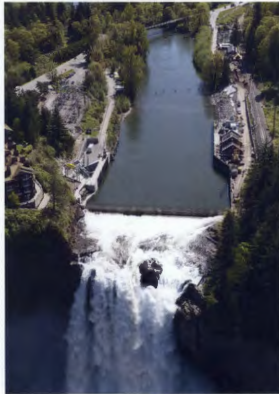
New intakes for the Snoqualmie Falls Hydroelectric facility can be seen on each side of the river above the falls.
