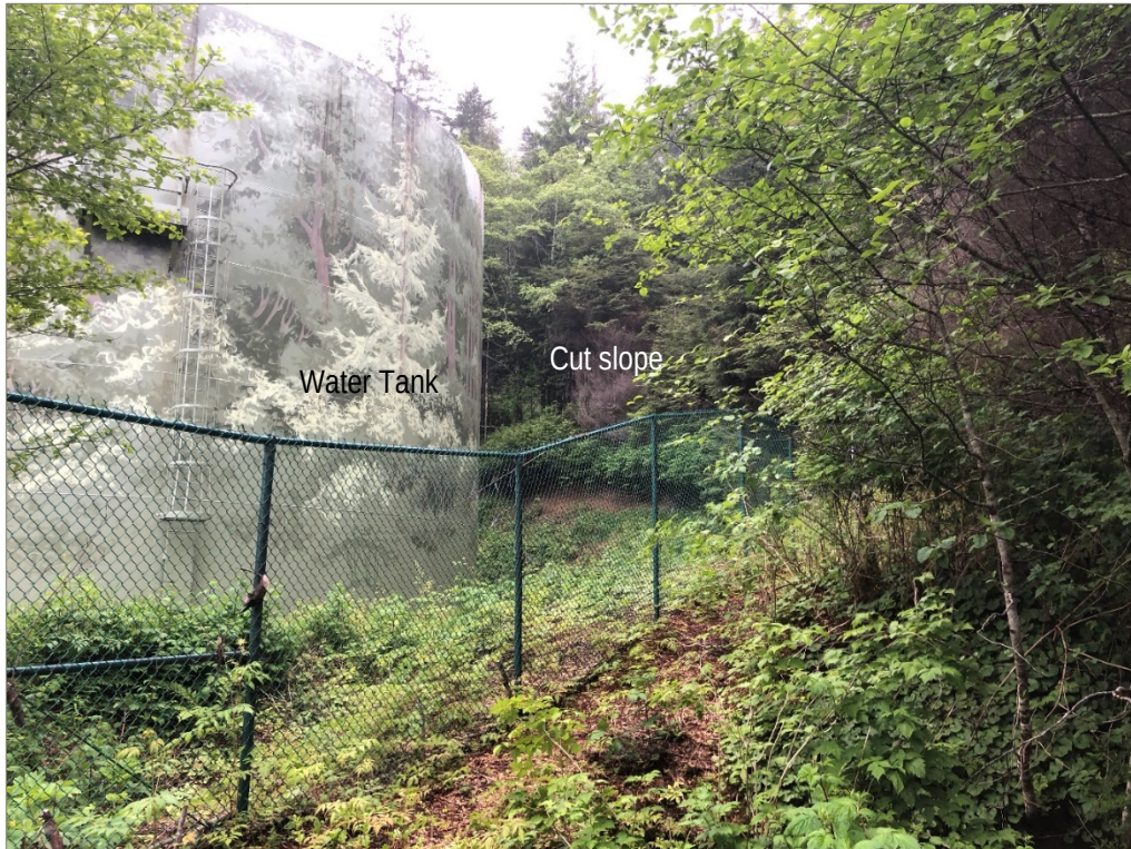
Exhibit 3-4: View to Northwest of Water Tank and Cut Slope
