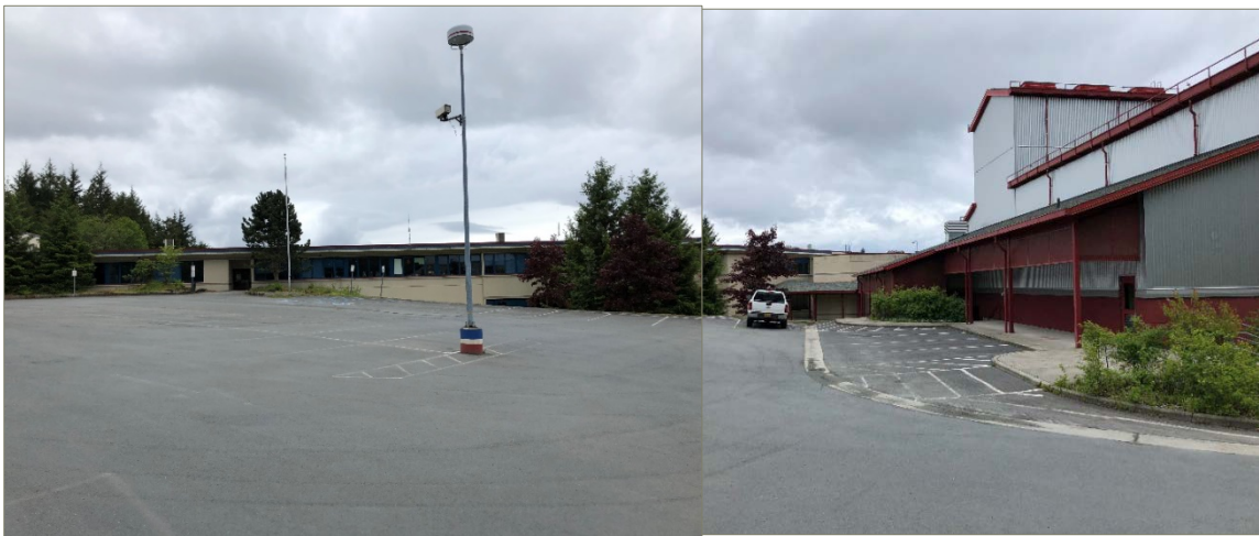
Exhibit 3-2: View South of the North-Facing Wall of the High School and Vegetated Terrain that is Upslope of Topographic Depression (Photo Left) and the Center for Performing Arts (Photo Right). Note the Distance Across the Parking Lot to the Wall of the High School Building that is Exposed to Potential Debris Flow Runout from Gavan Hill.
