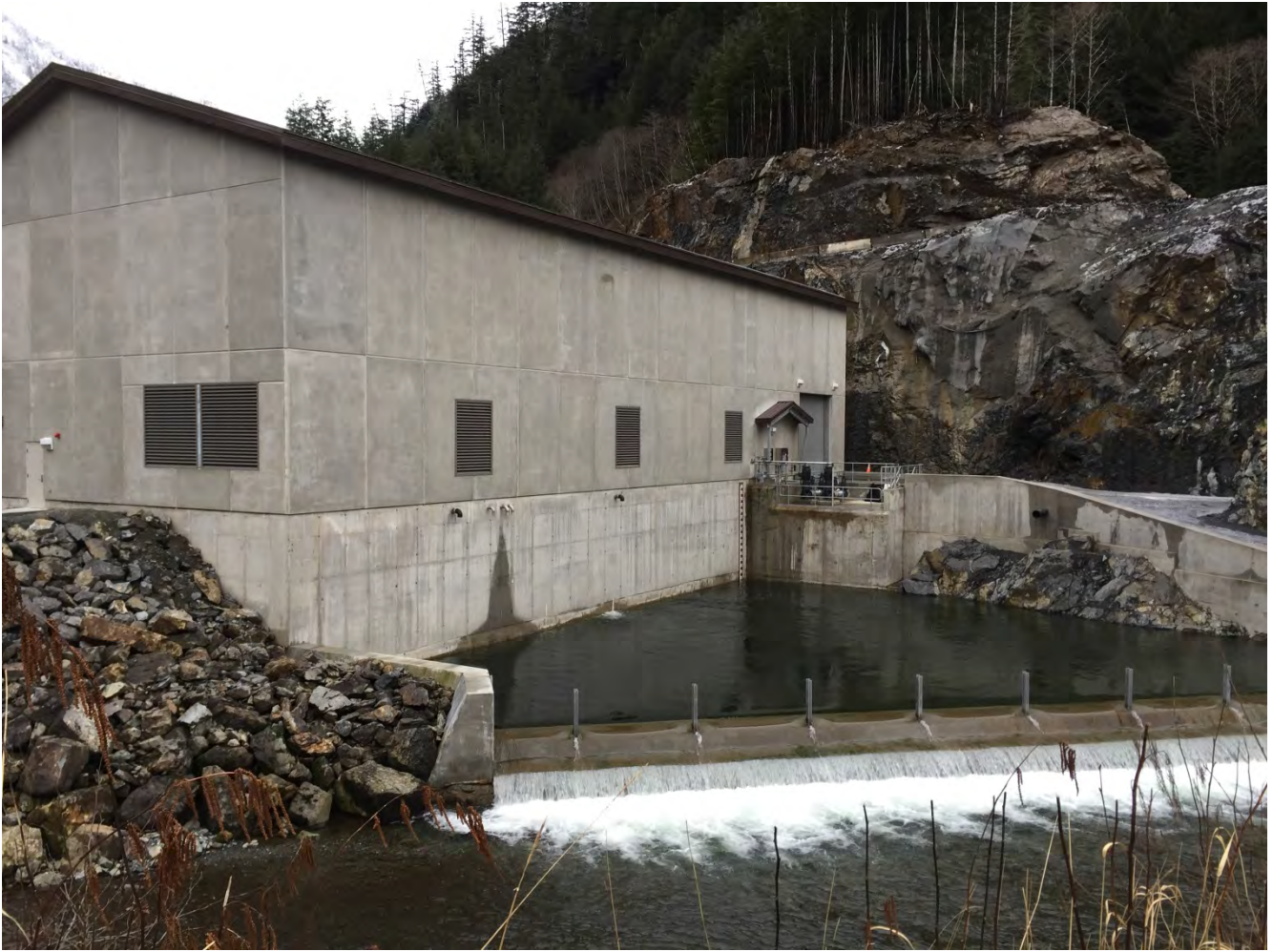
Figure 6. Powerhouse Site, no change this month.
