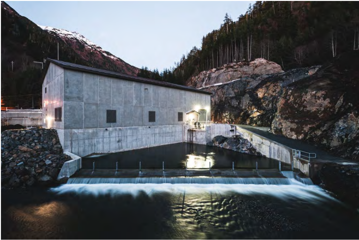
Figure 2: Powerhouse in Operation
