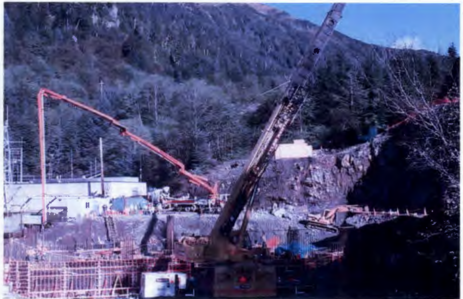
Crews work on the new Blue Lake powerhouse.
