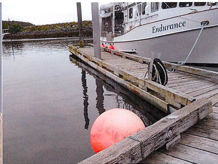
Showing loss of flotation in finger float, wood frame in contact with water
