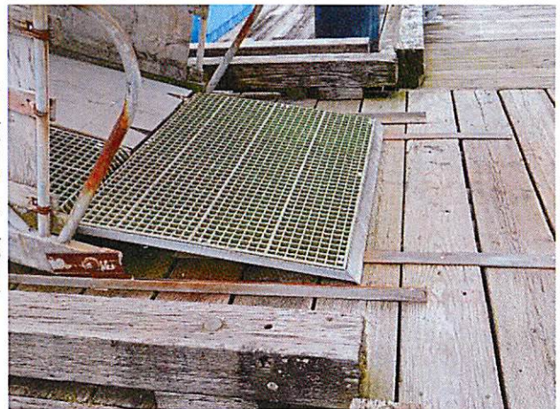
Trip hazard at gangway transition plate
