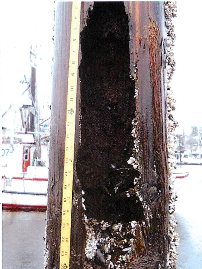
Extreme rot exhibited in timber piling. CBS has been methodically replacing timber piling as funding allows.
