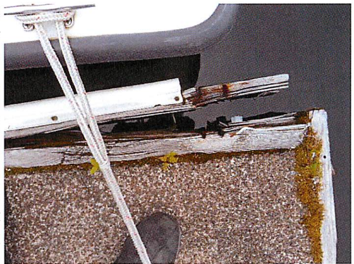
Damaged glulam
