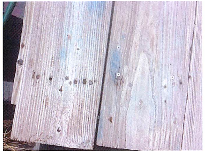
Staff have been forced to utilize multiple fasteners and ultimately transition from deck nails to screws to secure deck boards as a result of the rotten timbers sills and stringers
