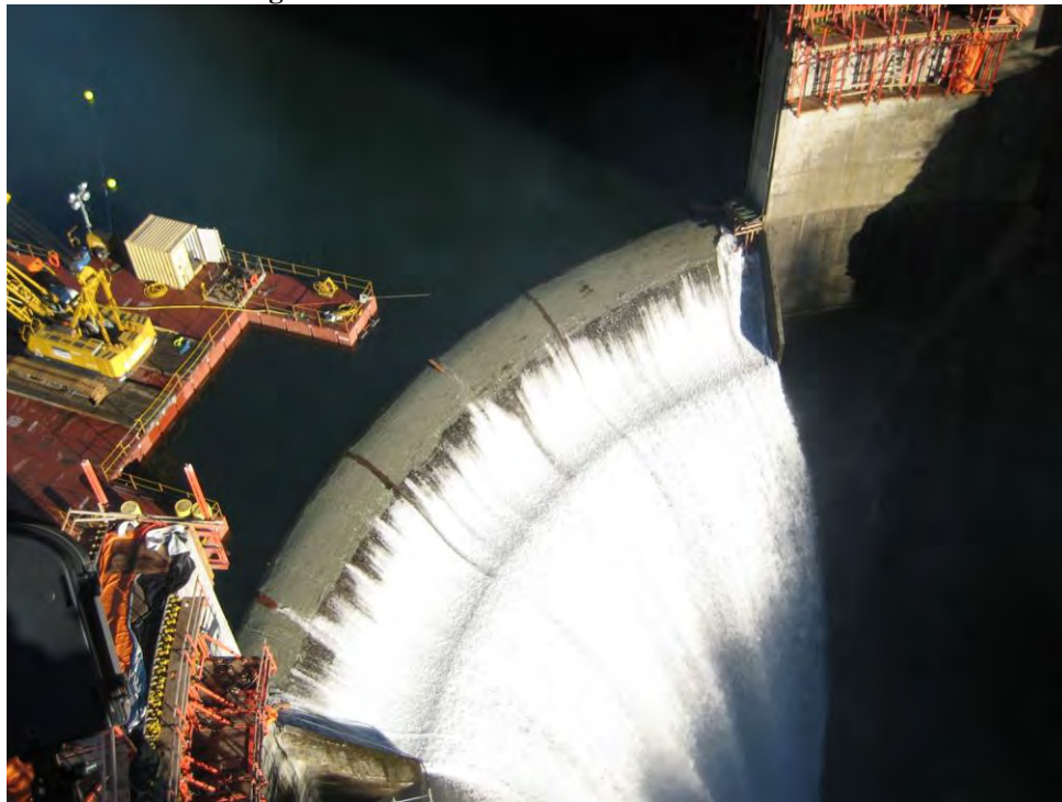
Figure 7: Blue Lake Spillway
