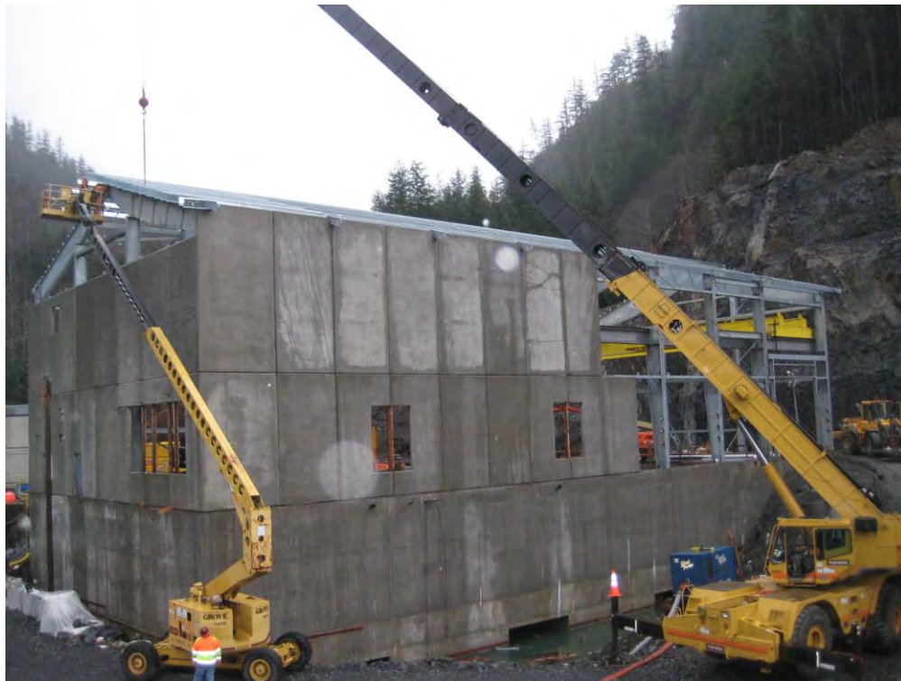
Figure 3: Precast Wall Panel Installation
