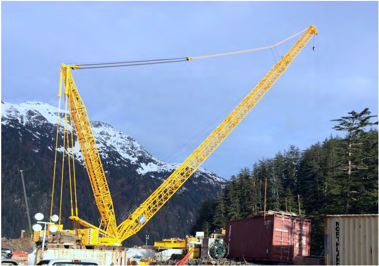
Figure 5. Dam Staging area, no change this month.
