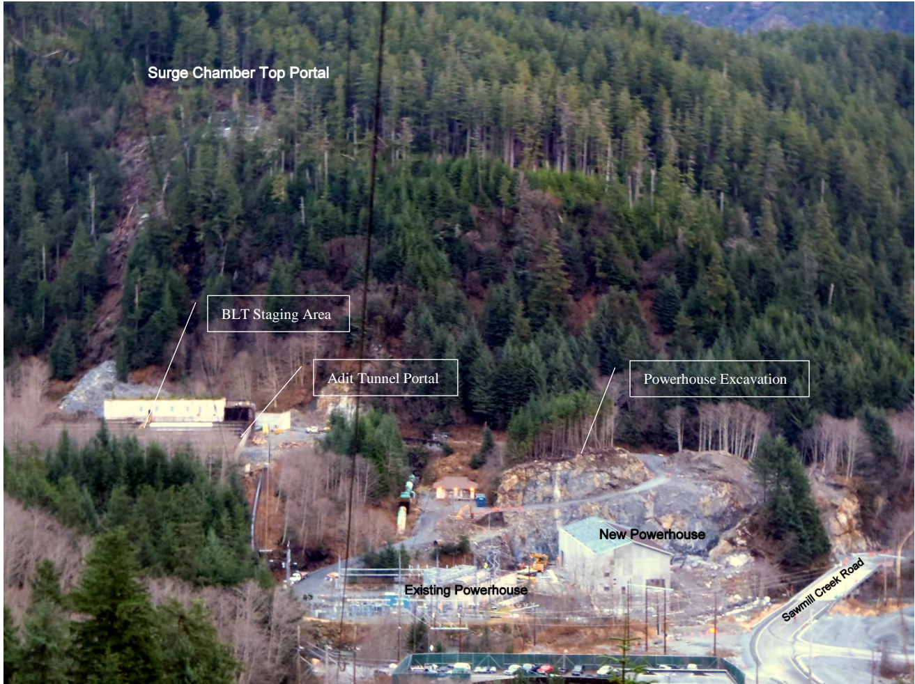
Figure 9. Lower Project Site, Southeast Earthmovers (SEEM) continued excavation on the new powerhouse access road.
