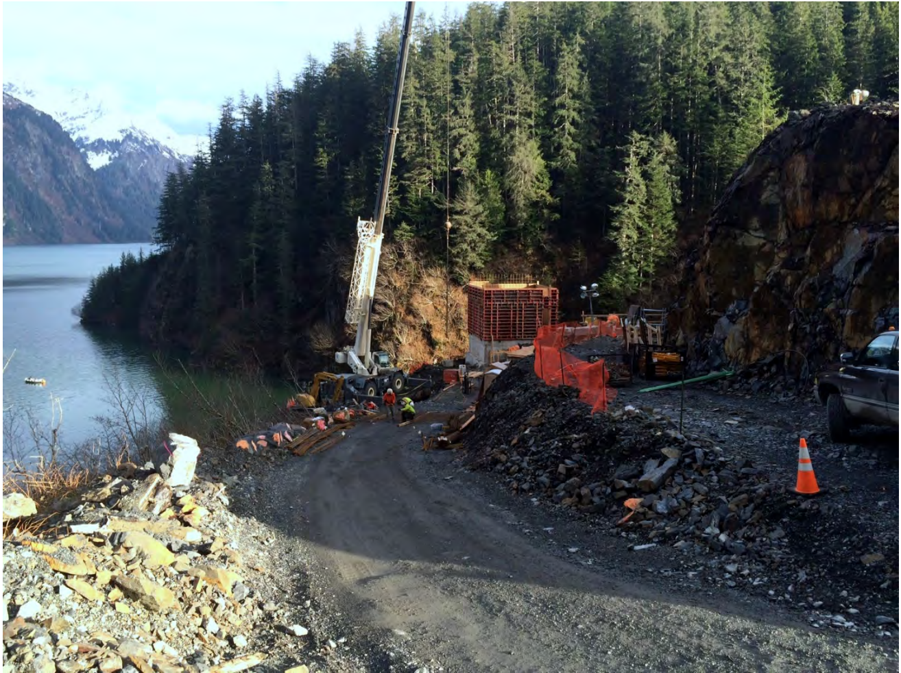
Figure 4. Gate House Location, Barnard made a gate house concrete floor placement and began working nightshift in the gate shaft installing gate guides.
