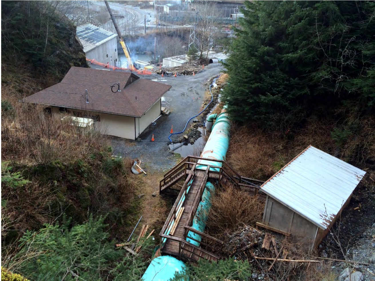
Figure 6. Lower Portal Area, no change this month.
