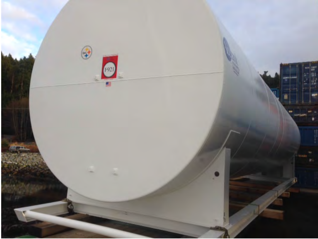
Figure 1. One of two 40,000 gallon above ground double-walled fuel tanks.
