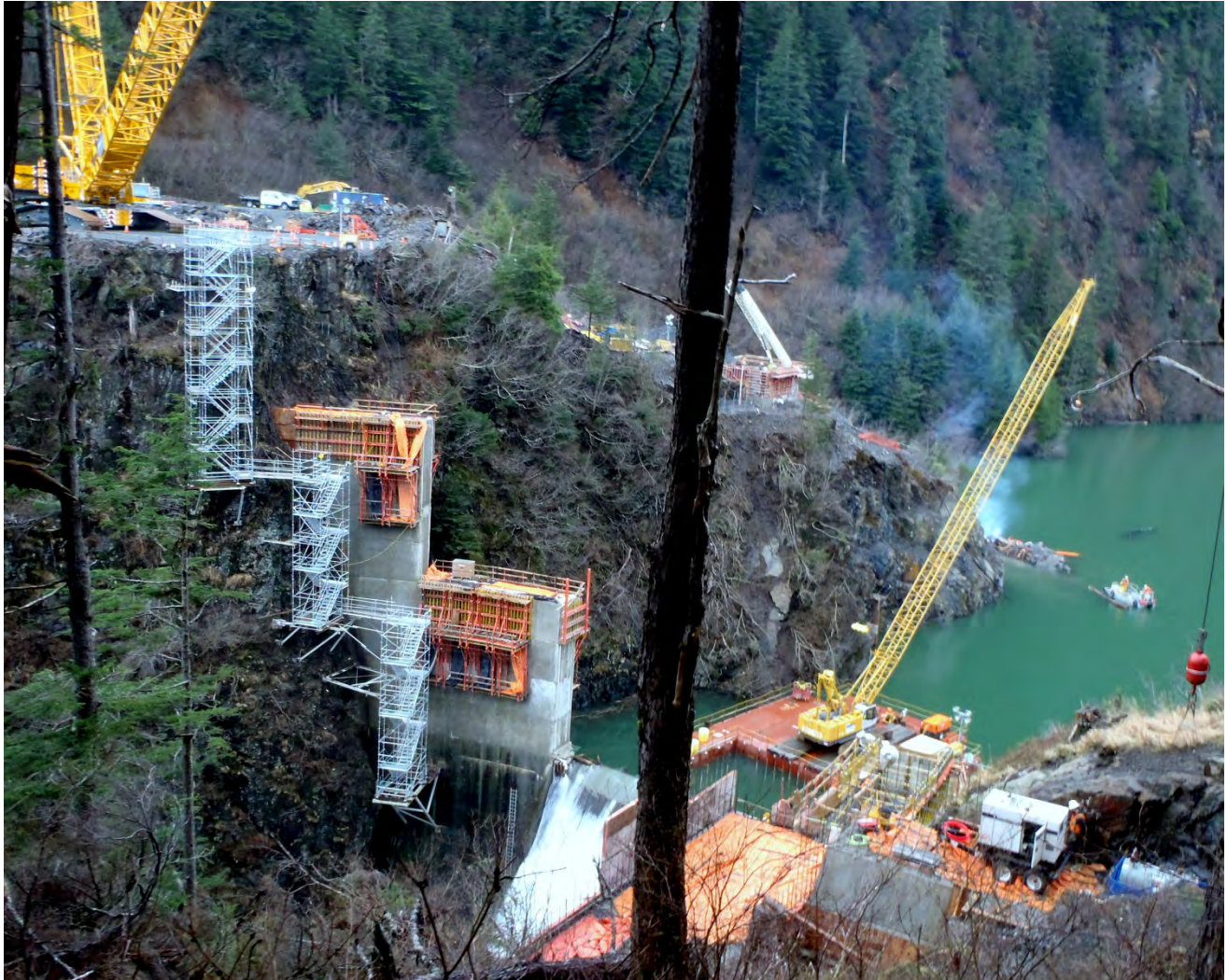
Figure 3. Intake Portal and Right Abutment, Gatehouse foundation is complete.
