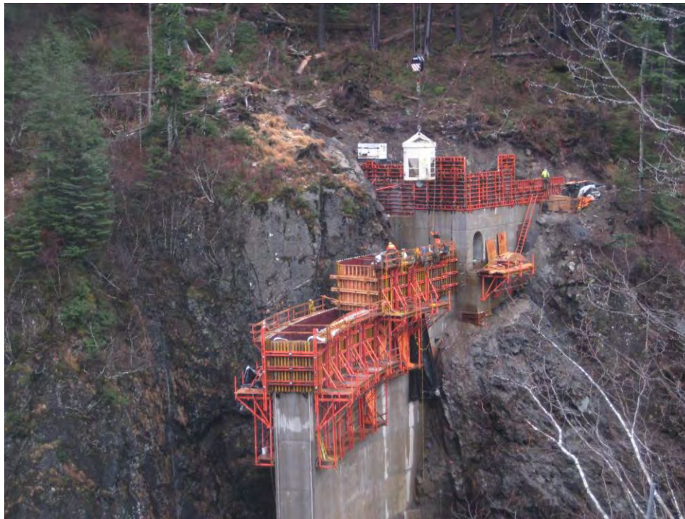
Figure 5: Concrete Placement for M7-403
