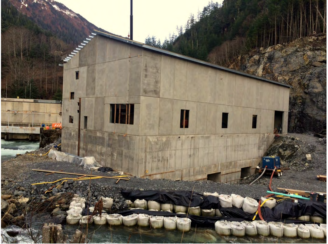
Figure 7. Powerhouse Site, ASRC McGraw Constructors (AMCL) completed the installation of the concrete wall panels and began the installation of the roof panels.
