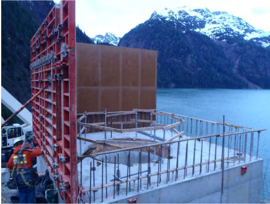
Figure 6: Gatehouse Floor and Wall Formwork
