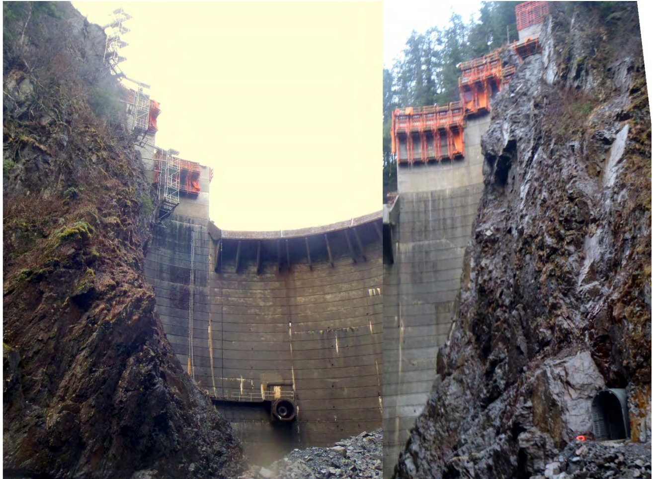
Figure 2. Drainage Tunnel and Scour Wall, on January 29 the lake stopped spilling.
