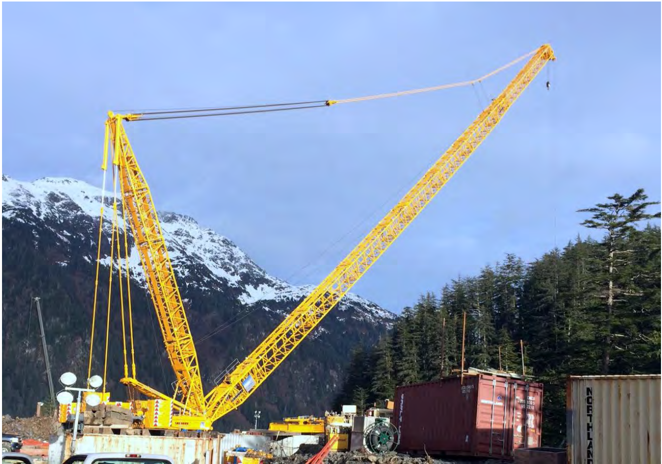
Figure 5. Dam Staging area, no change this month.
