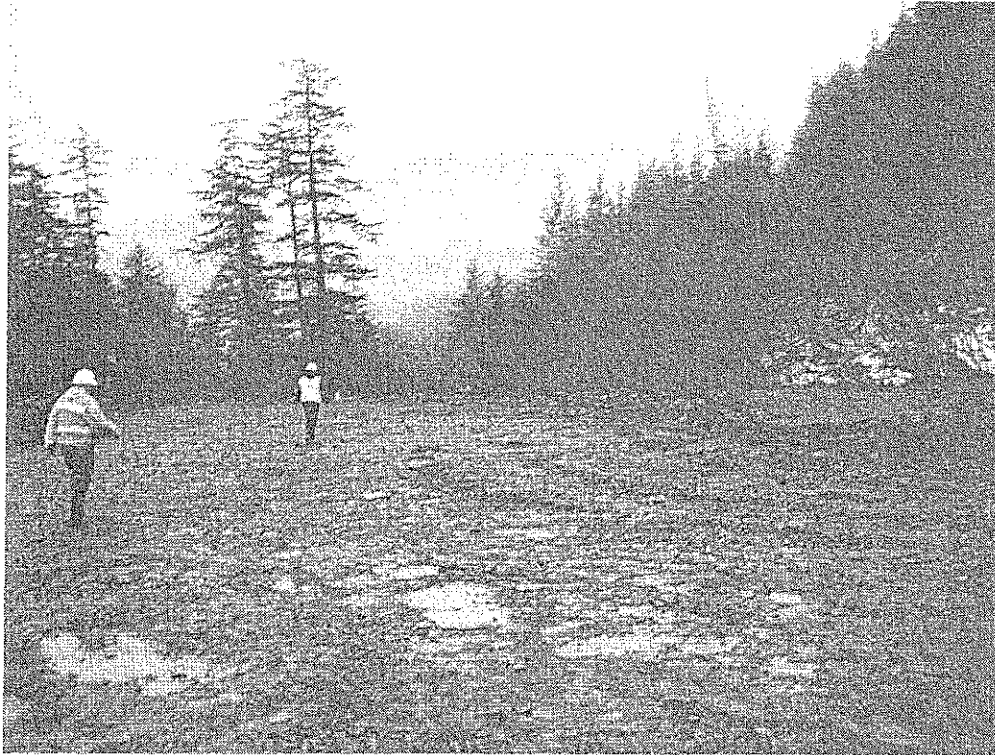
Figure 2: Dam Staging Area - Late January
