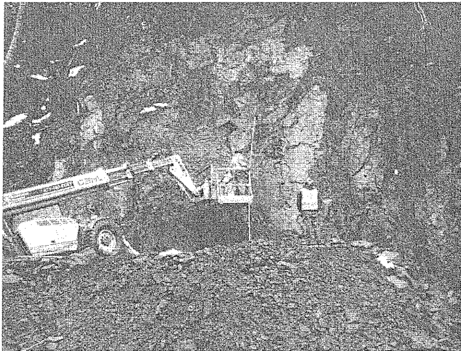
Figure 5: Adit Tunnel Portal Rock Support
