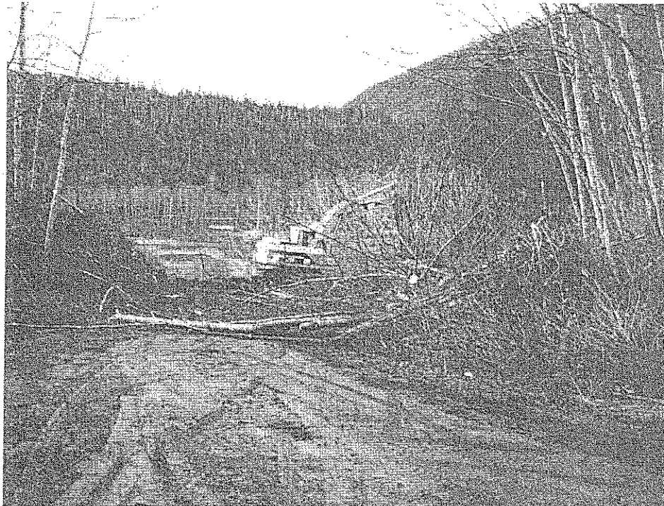
Figure 3: Powerhouse Access Road Clearing
