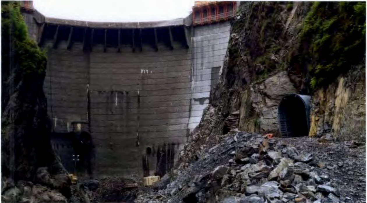
Figure 2. Drainage Tunnel and Scour Wall, the lake finished spilling.
