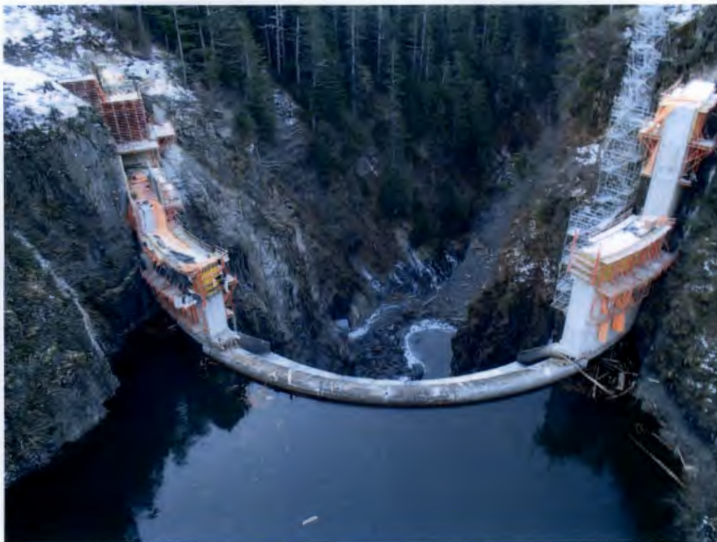
Figure 2: Bird's Eye View of Dam Raise
