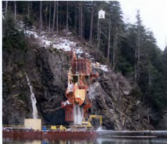
Figure 1: Left Abutment Dam and Thrust Block
