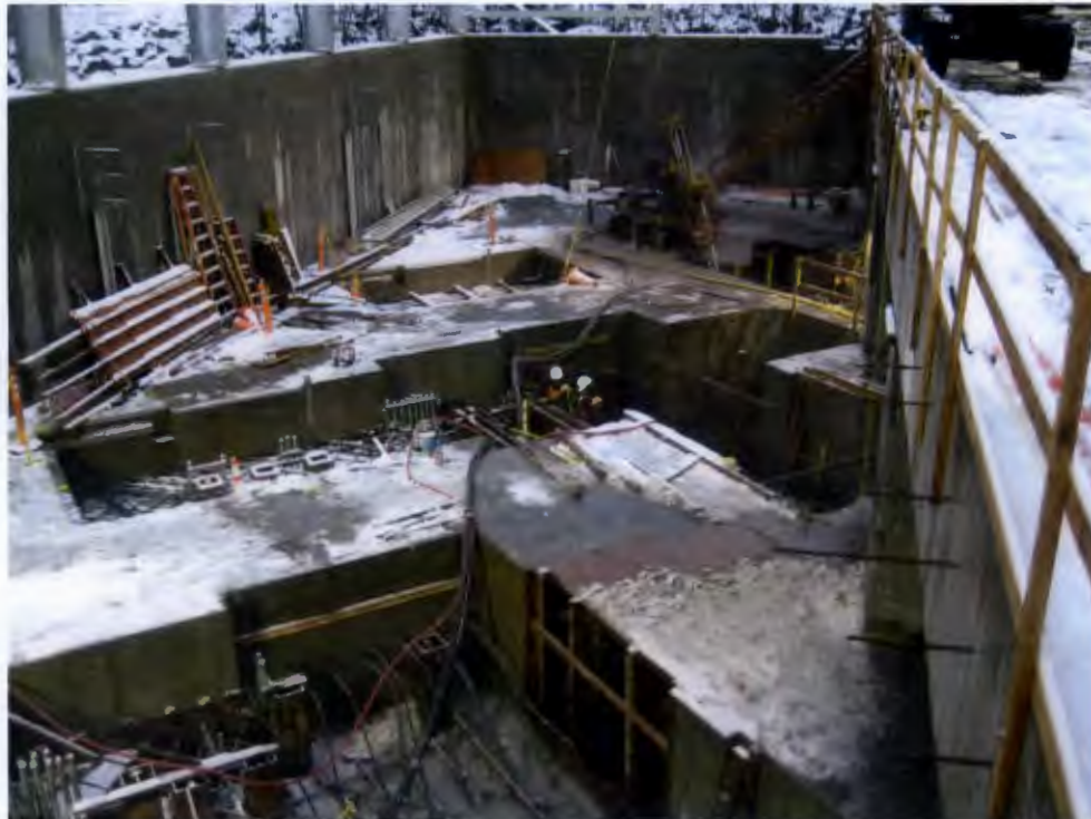
Figure 4: Powerhouse Turbine Pits
