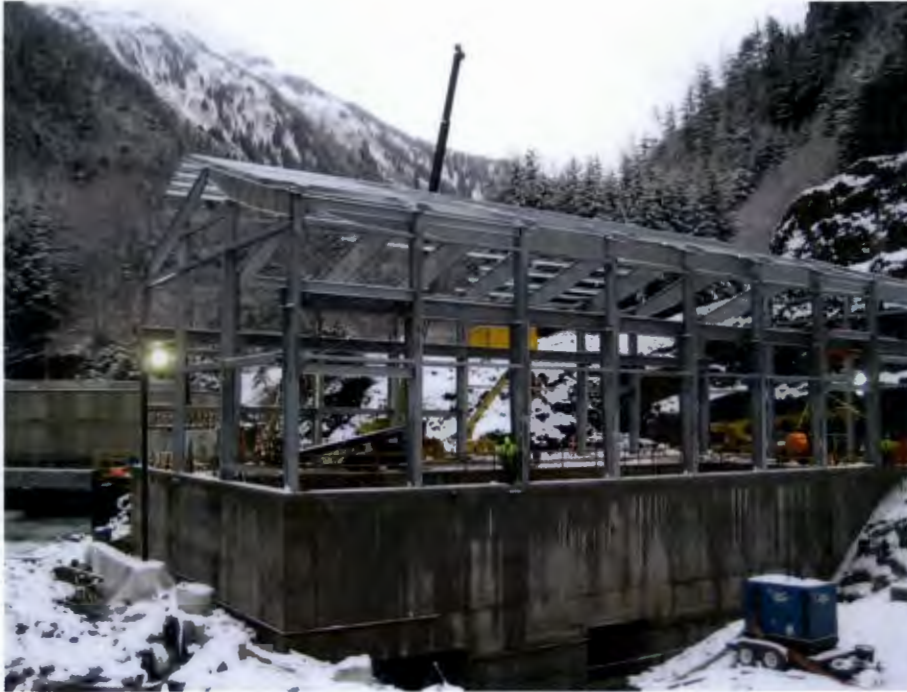
Figure 3: Powerhouse Steel Building
