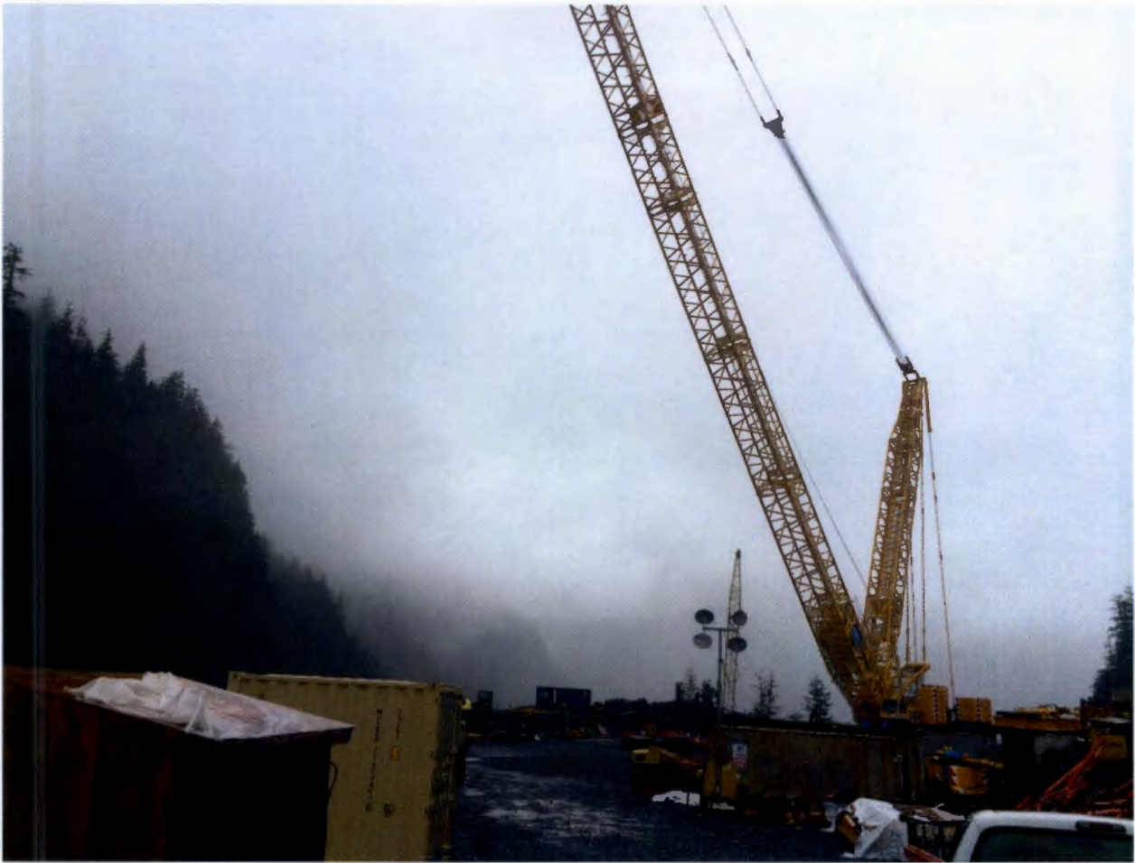
Figure 5. Dam Staging area, No change this month.
