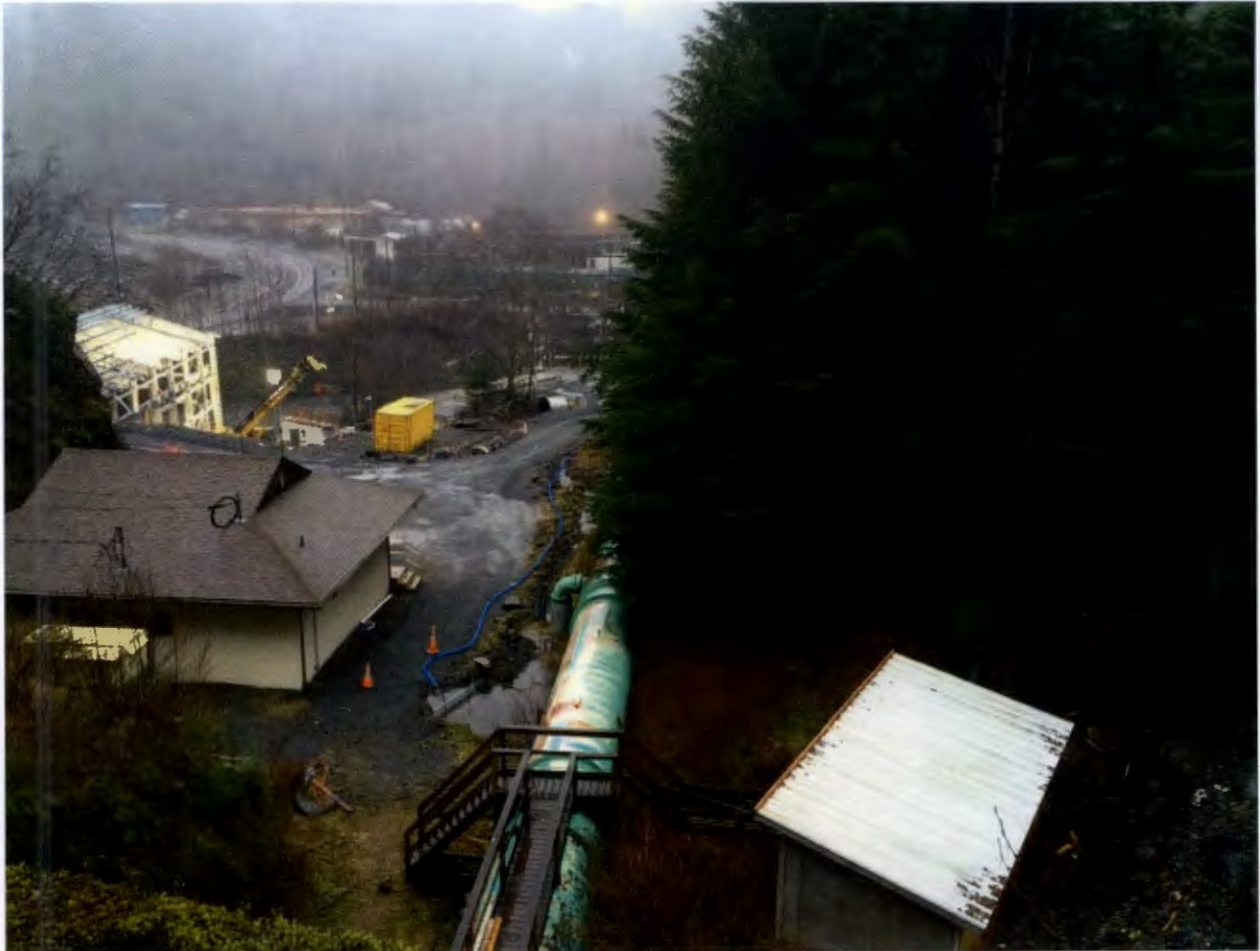
Figure 6. Lower Portal Area, no change this month.
