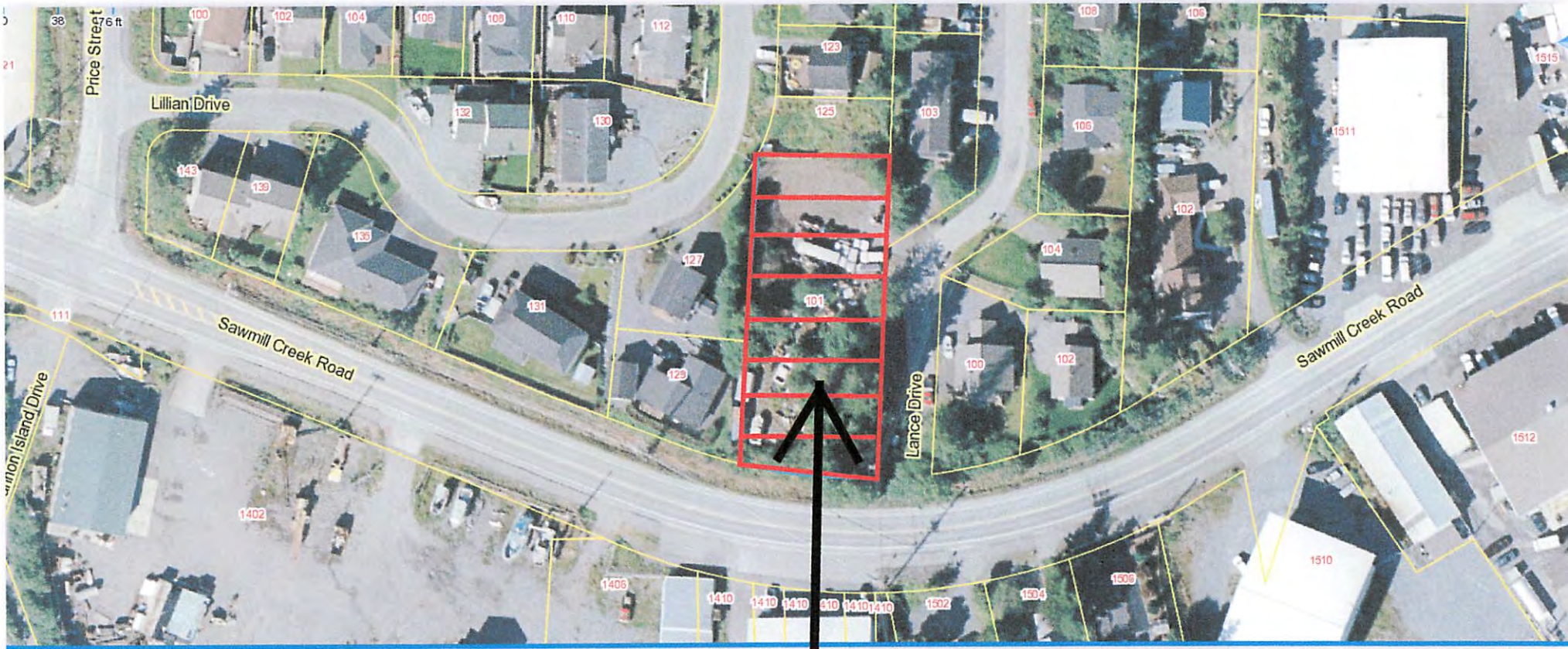
Burkhardt Zoning Violation 101 Lance Drive
