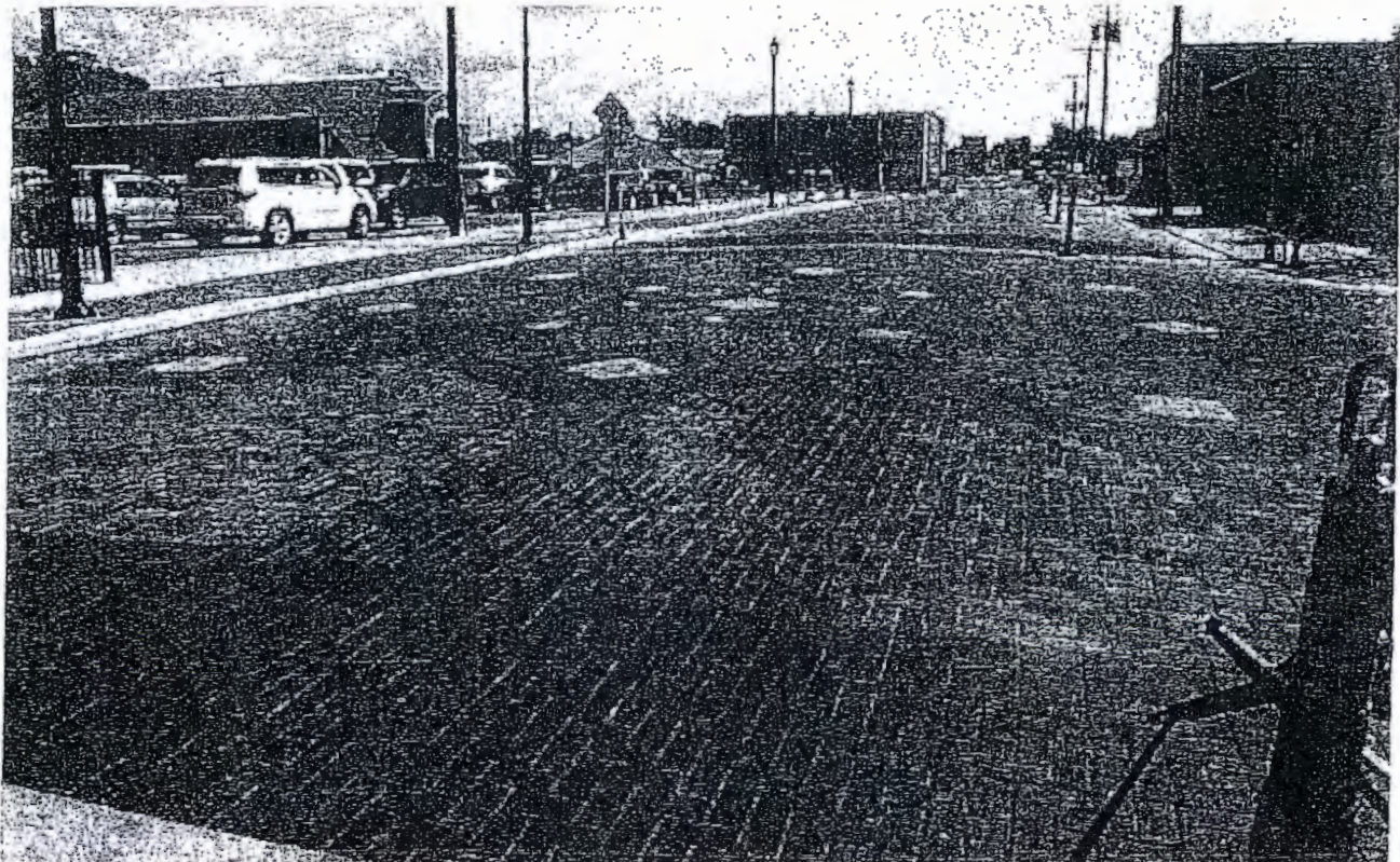
An example of how new hardscape can enhance public space.
