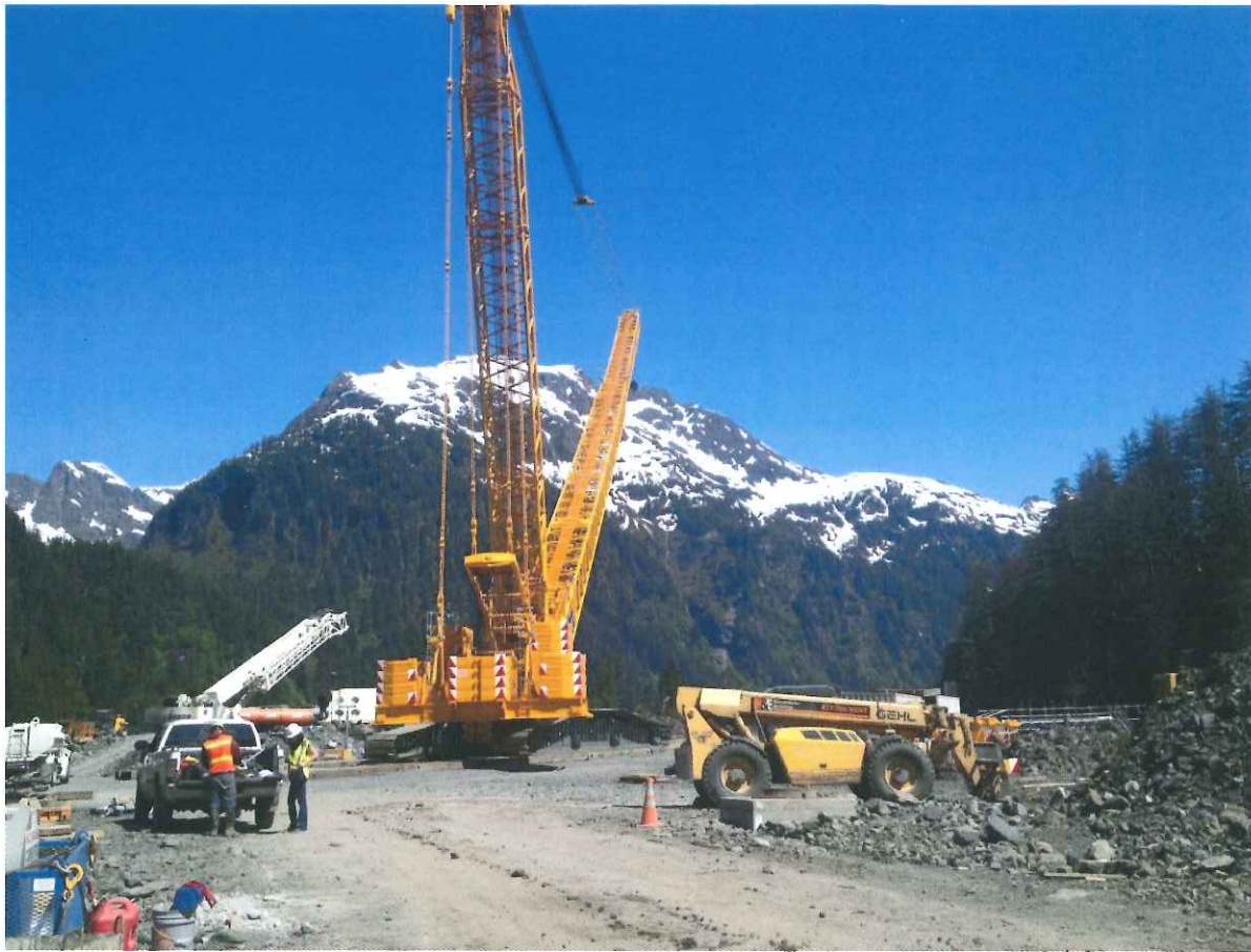
Figure 5. Dam Staging area, Continued use of the staging area for both cranes and eventually tunnel muck from the intake excavation will be stored here.
