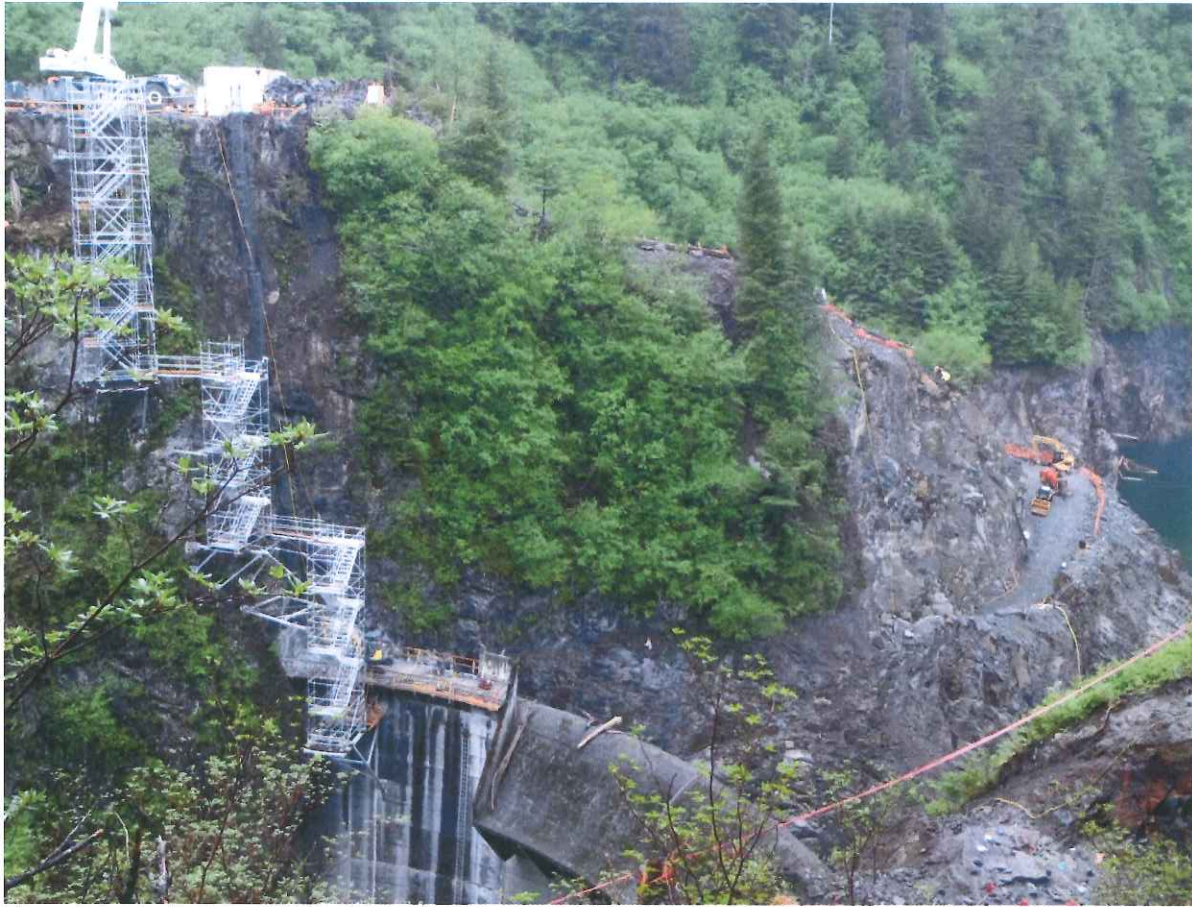
Figure 3. Intake Portal and Right Abutment, – Excavation along the tunnel intake access road reached the intake portal location (the face of the tunnel entrance). Blue Lake Tunnelers is now working 24/7 with two crews to excavate the intake tunnel. Scaffolding was erected to reach the top of the dam from the staging area to prepare the right abutment for the dam raise.
