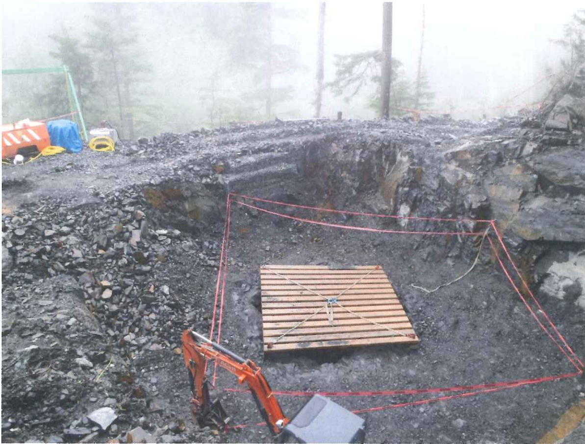
Figure 6. Surge Chamber Top Portal, Work to prepare the top portal for the small structure that will be constructed over the opening is complete.
