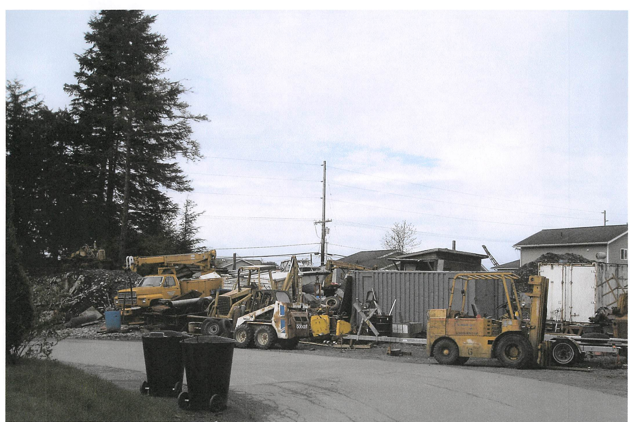
101 Lance Drive Pictures of property 4/30/15
