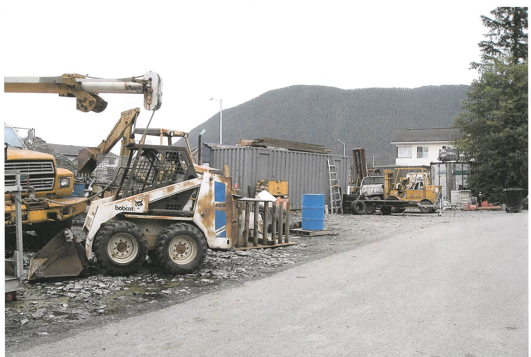
101 Lance Drive Pictures of property 7/1/15
