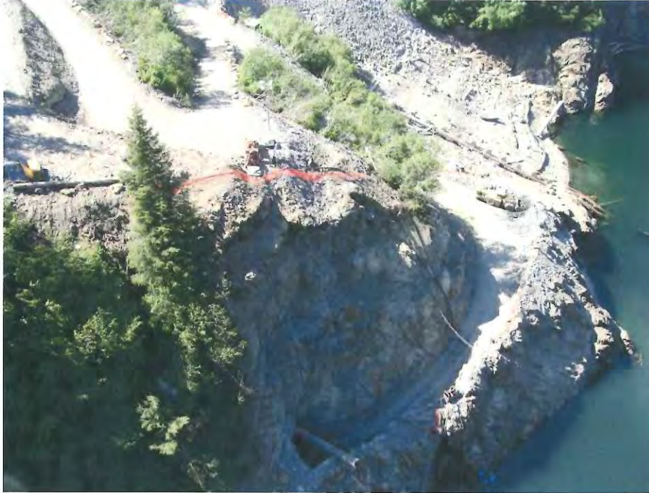
Figure 2: Aerial View of Intake Tunnel Portal
