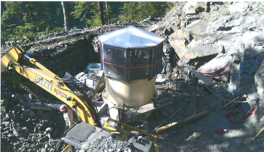
Figure 3: Surge Shaft Top Structure
