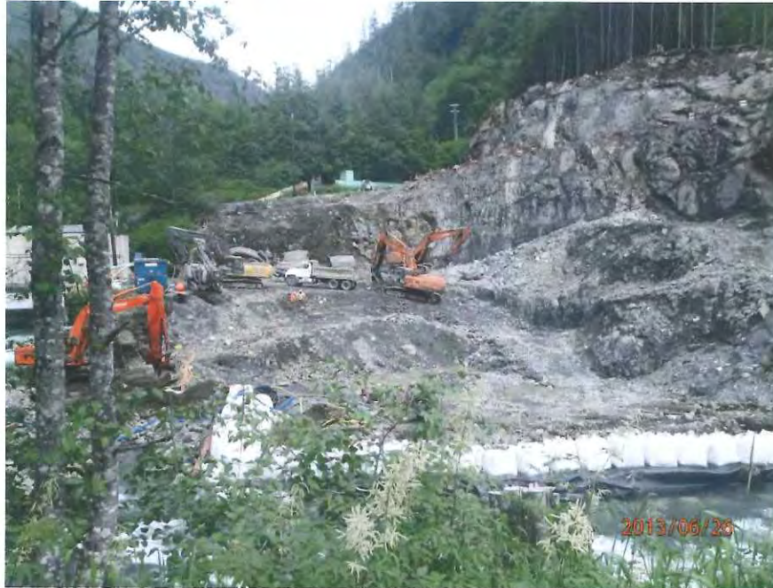
Figure 4: Powerhouse Excavation
