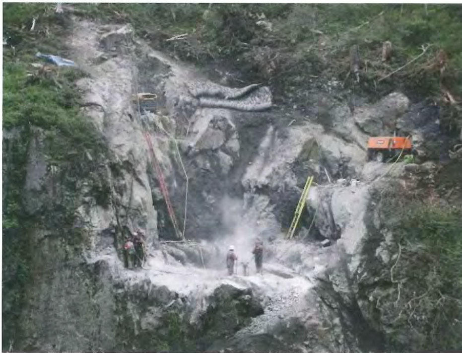
Figure 1: Left Abutment Excavation
