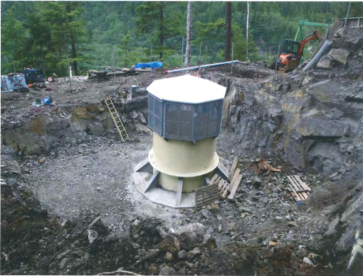
Figure 6. Surge Chamber Top Portal, The small structure over the surge shaft is complete.
