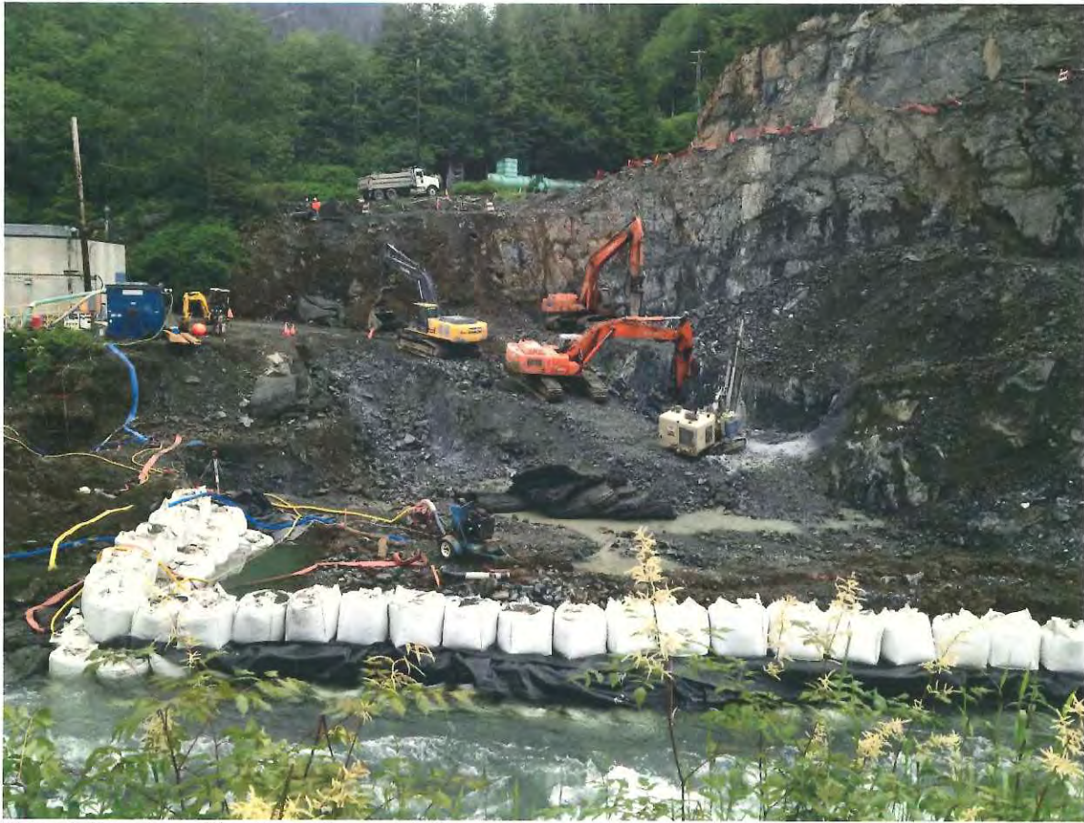
Figure 8. Powerhouse Site, Excavation work in the powerhouse area continued all month with additional work shifts added.
