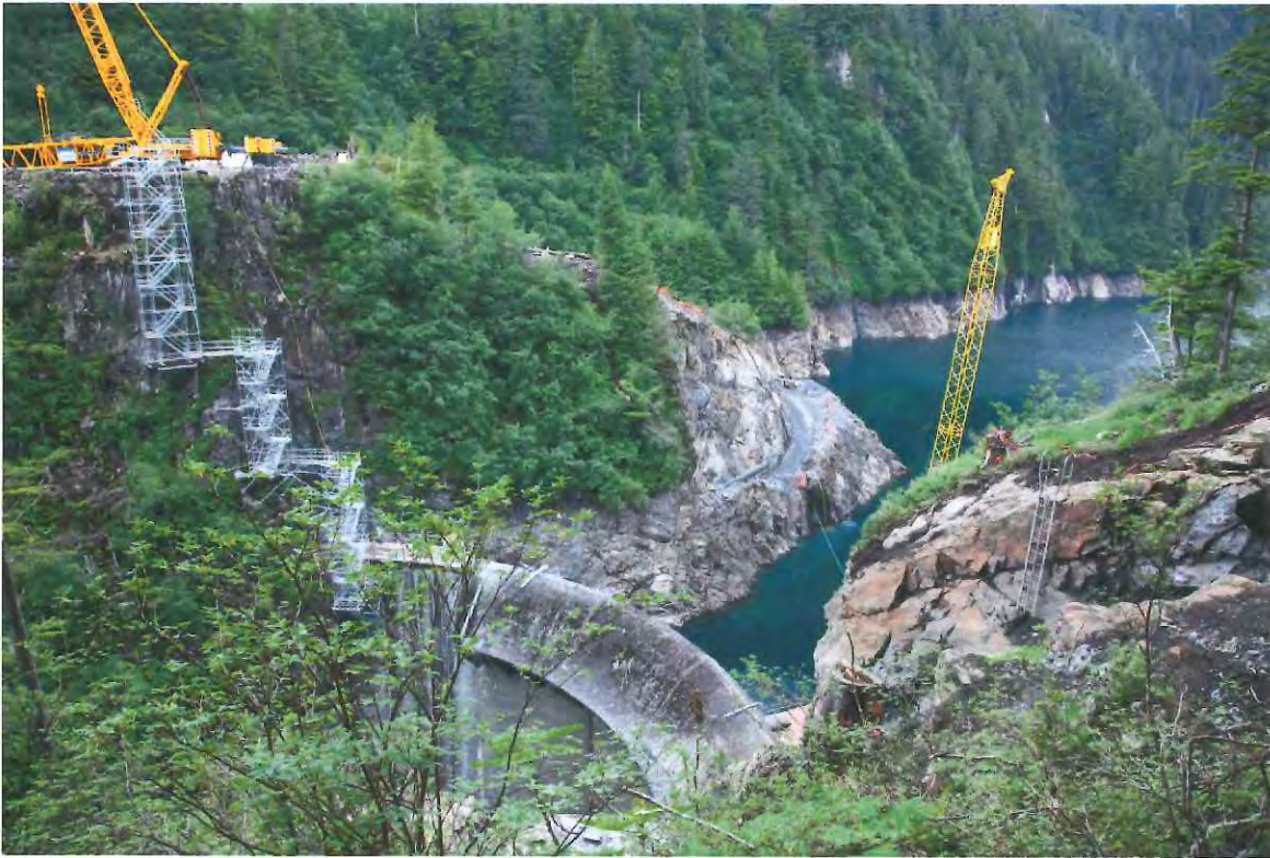
Figure 3. Intake Portal and Right Abutment, Blue Lake Tunnelers have completed 700 of 829 feet of the intake tunnel.
