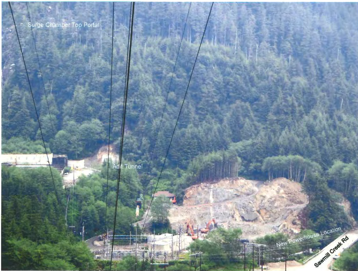
Figure 8. Lower Project Site, Excavation of the new powerhouse site is ongoing.
