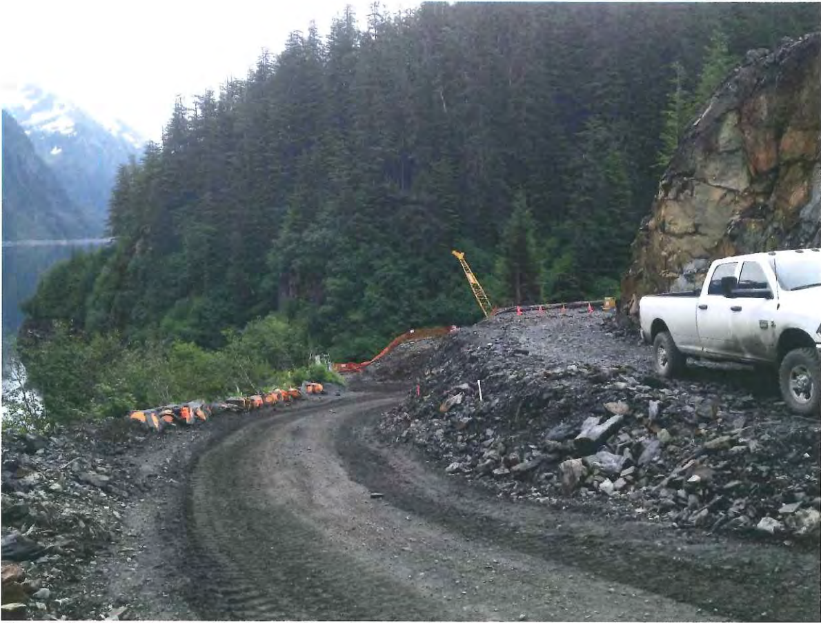
Figure 4. Gate House Location, No change this month.
