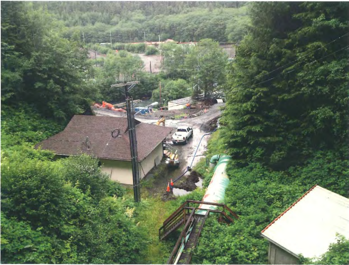
Figure 7. Lower Portal Area, No change this month.
